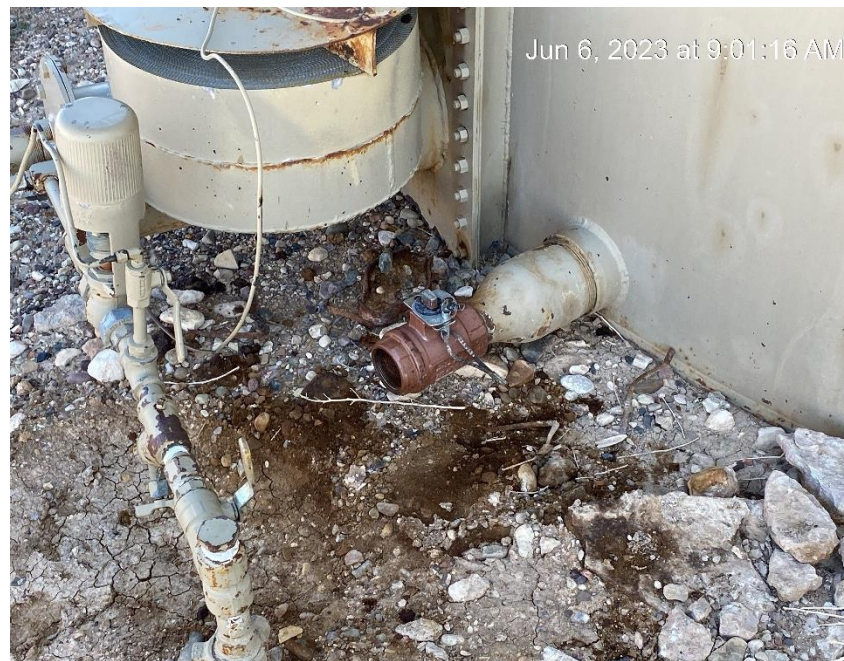
Open end tank valve. Stained soil
