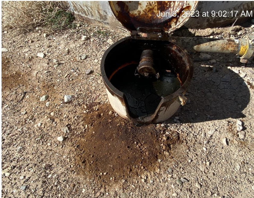
Full of oil and leaking. Stained soil
