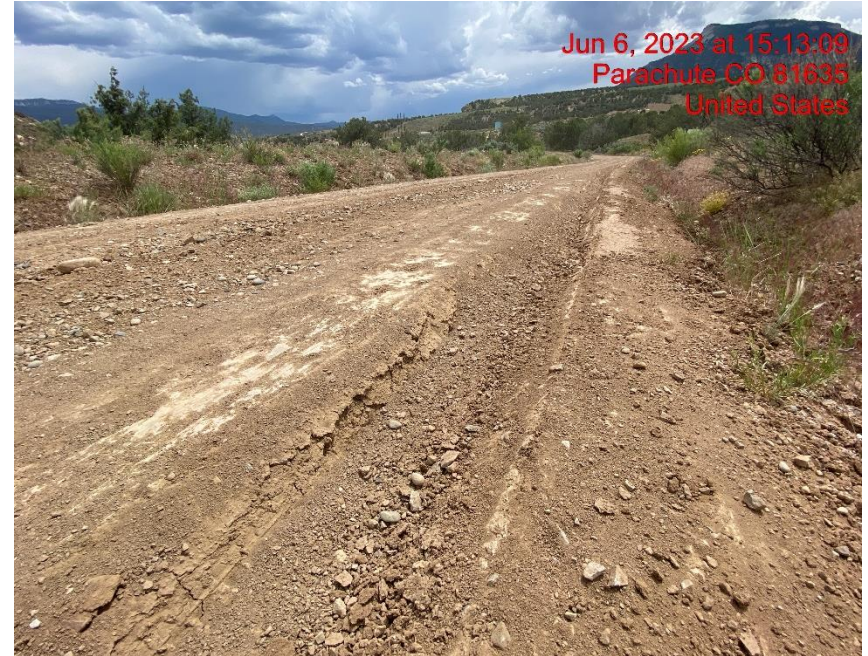
Lease Road Lacks Stabilization – Photo #04212
