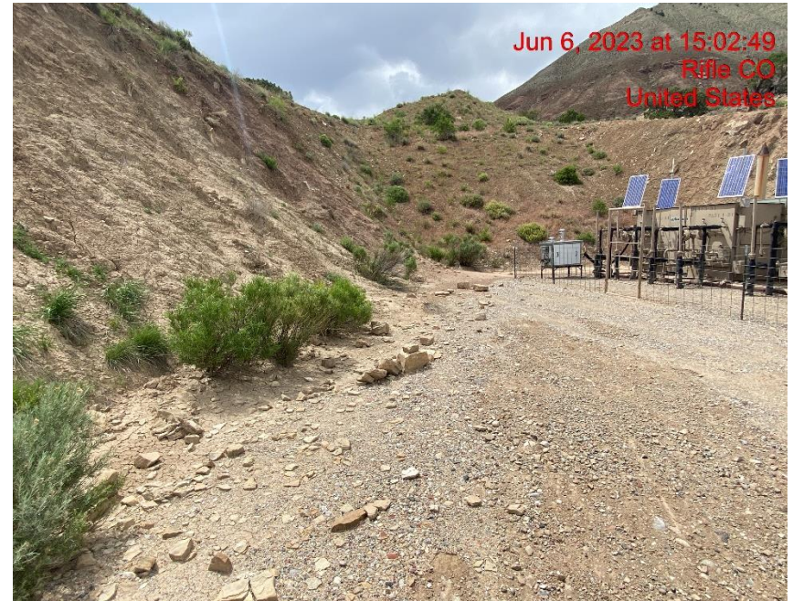
Cut Slope Eroding onto Location – Photo #04201
