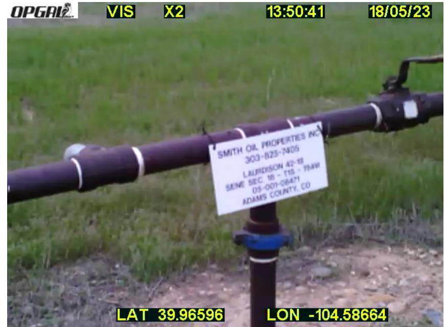
Photo# 4 leak at well head.
