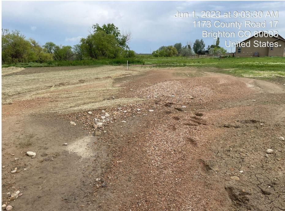
**Photo 3. Photo taken of sediment accumulation from stormwater flowing over the site.**
