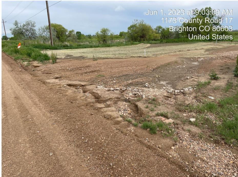
**Photo 1. Photo taken of stormwater erosion along country road onto site.**
