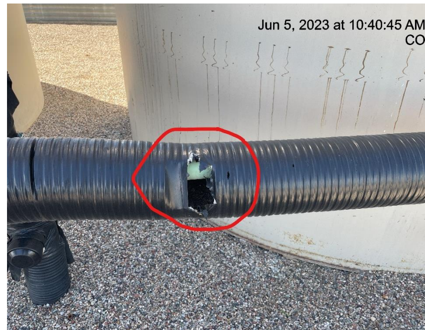
Photo # 9414 Hole in flowline heating insulation/wildlife hazard
