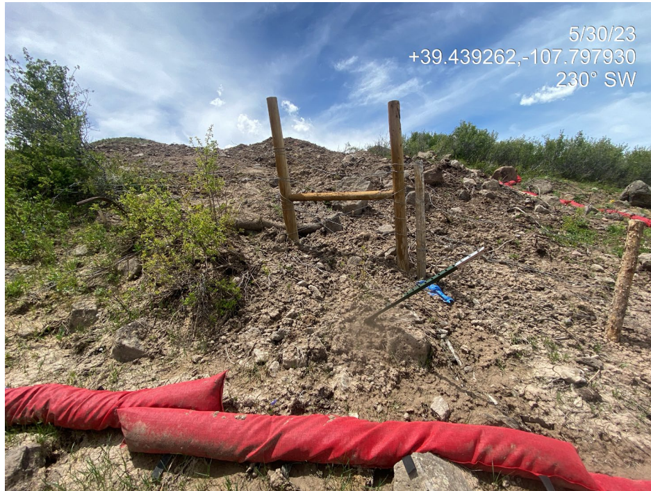
Photo 14. Photos show lack of stabilization BMPs on soils at the east of the location. Sediment is accumulating downslope, offsite.
