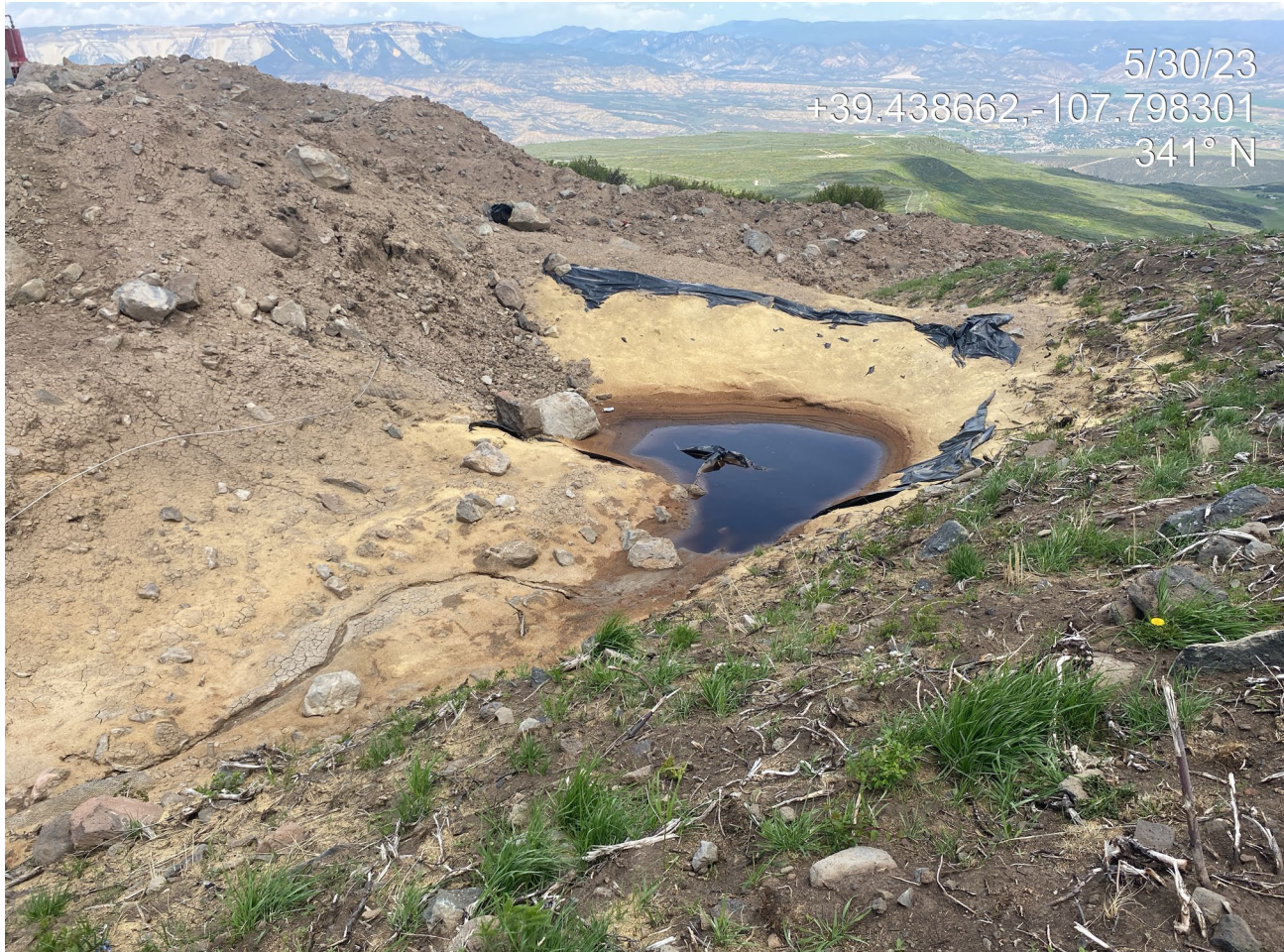
Photo 4. Photo taken from the southeast shows the topsoil stockpile (right) is not properly segregated from subsoils and possible cutting trench materials. The liner pictured is in disrepair. A straw wattle at the base of the topsoil stockpile is not present in areas adjacent to the cuttings trench.
