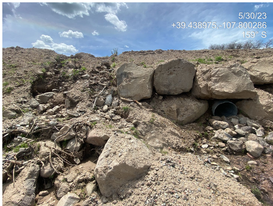
Photo 21. Photos taken from the access road to the west of the location. Stormwater is bypassing a culvert and eroding the road fill (left) and overtopping wattles, and transporting and depositing sediment in undisturbed areas offsite (right).
