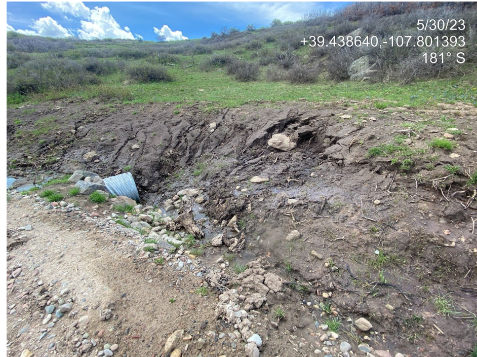
Photo 23. Photos show sloughing, slumping and rill erosion occurring on the access road cut.
