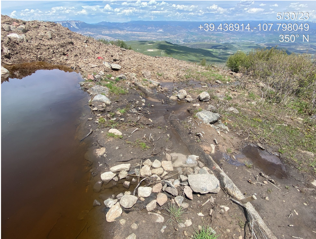
Photo 10. Photo shows a sediment trap at the northeast. The outlet is degraded and eroded and appears to have lost rip-rap. Sediment laden stormwater is exiting the trap in multiple places without a properly engineered outlet.
