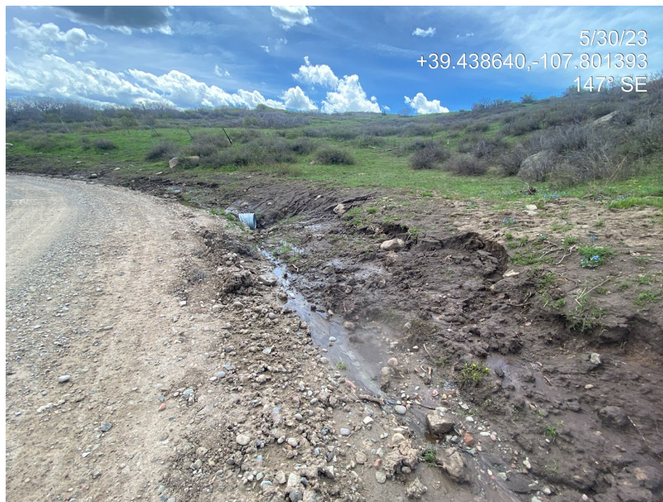
Photo 23. Photos show sloughing, slumping and rill erosion occurring on the access road cut.
