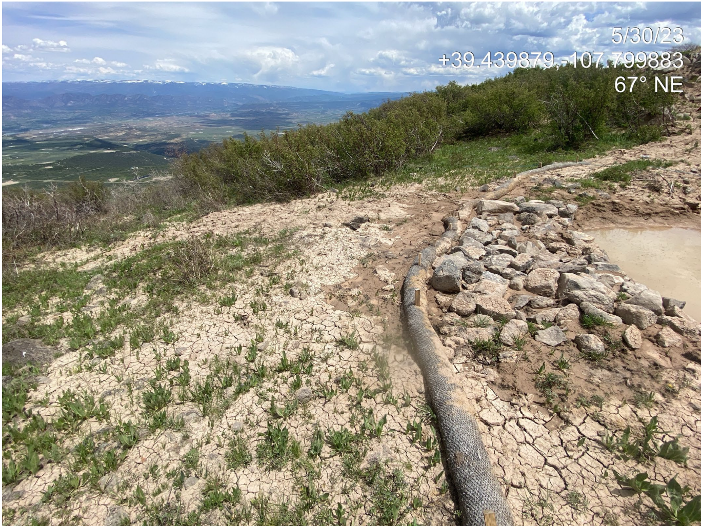
Photo 19. Photo shows sediment laden stormwater bypassing a sediment trap outlet resulting in offsite degradation and sediment transport.
