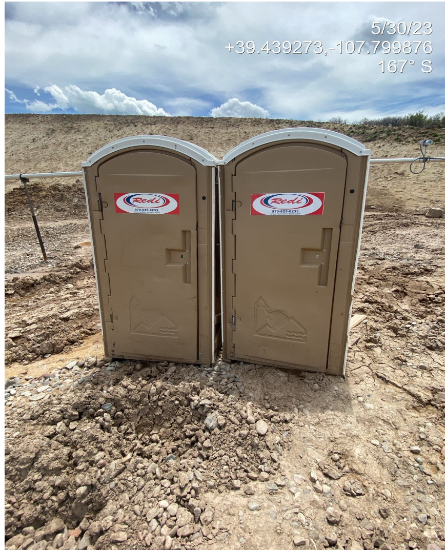
Photo 7. Photo taken from the Location entrance shows portable toilets have not been secured to prevent a spill.
