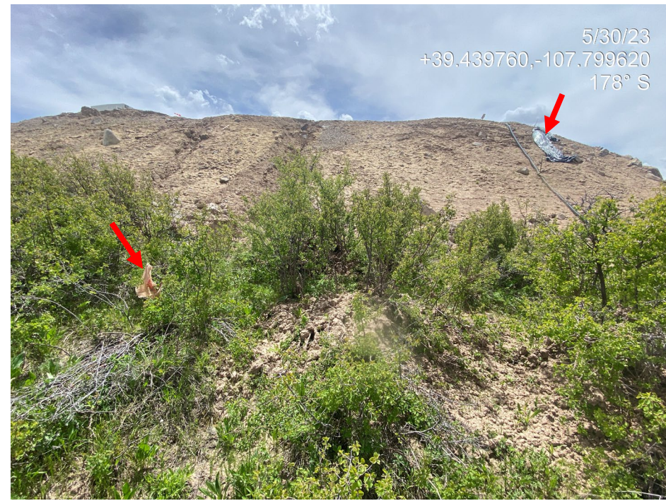
Photo 18. Photos show offsite sediment transport below the fill slope gullies pictured on the previous slide. Note also trash/debris (arrows).
