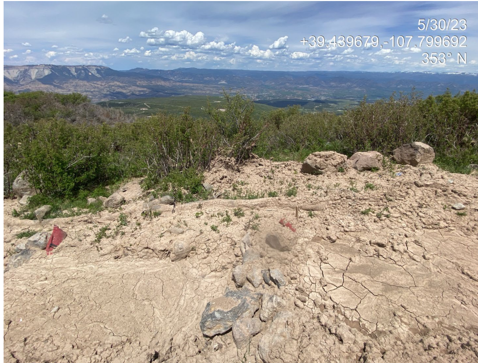
Photo 18. Photos show offsite sediment transport below the fill slope gullies pictured on the previous slide. Note also trash/debris (arrows).
