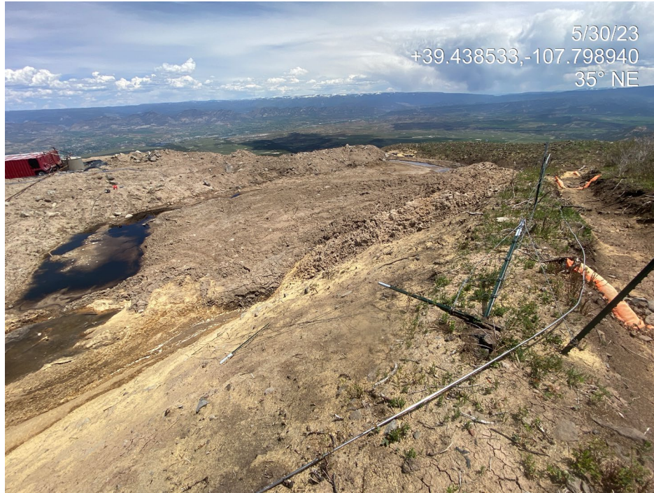
Photo 2. Photos taken from the south show an overview of the western (left) and eastern (right) portions of the cuttings trench. Trench perimeter fencing is in disrepair and non-functioning.
