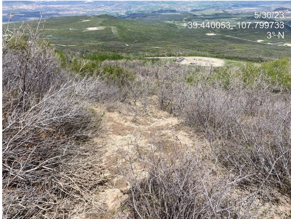
Photo 20. Photos show offsite sediment transport below the sediment trap pictured on the previous slide.
