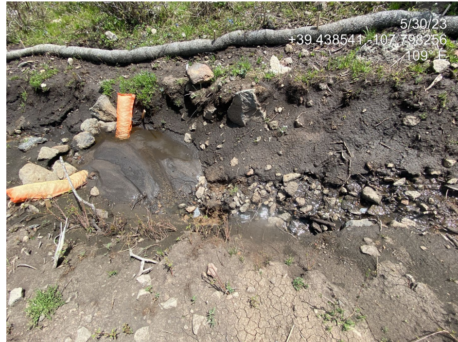
Photo 8. Photos show scouring and rill erosion in the eastern perimeter stormwater ditch resulting in degradation to the BMP and increased sediment loads. Sediment has filled in the check dam.
