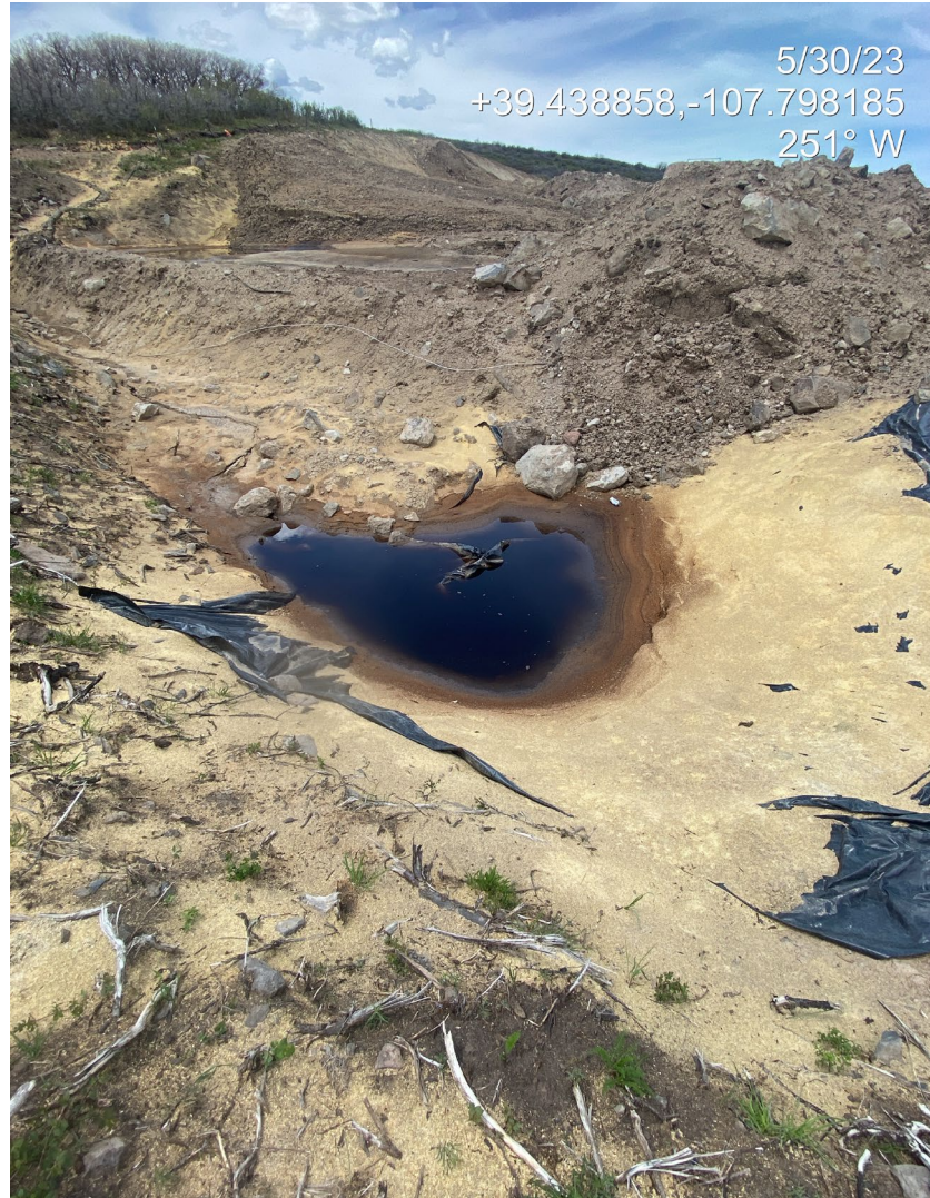
Photo 5. Photo taken from the southeast shows the topsoil stockpile (left) is not properly segregated from subsoils and possible cuttings trench materials. The liner is in disrepair. A straw wattle at the base of the topsoil stockpile is not present in areas adjacent to the cuttings trench.
