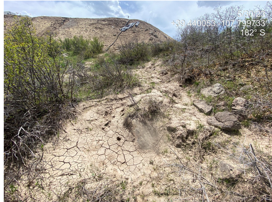
Photo 20. Photos show offsite sediment transport below the sediment trap pictured on the previous slide.
