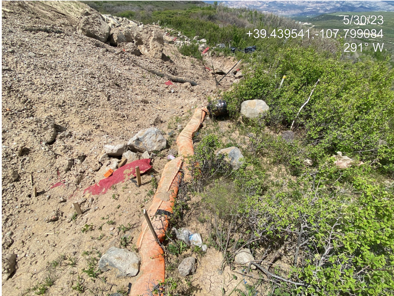
Photo 16. Photo shows the perimeter stormwater ditch to the northwest is filled with eroded fill material and no longer functioning as a ditch to properly transport water. Note also trash.
