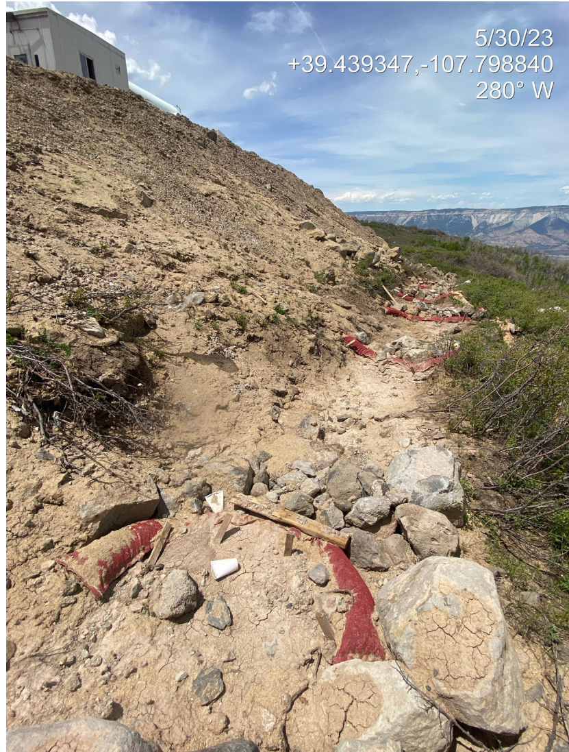
Photo 15. Photo shows sediment deposition downslope of the northern perimeter stormwater ditch. Stormwater is exiting the ditch in multiple places. The ditch is filled with sediment. Note also trash.
