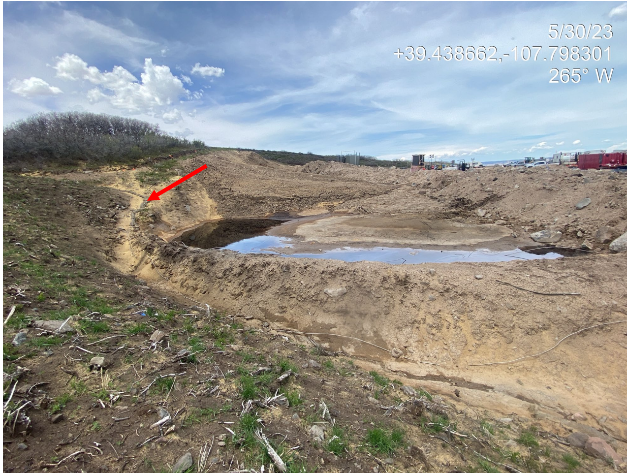
Photo 6. Photo taken from the southeast shows the topsoil stockpile (left) is not properly segregated from subsoils and possible cutting trench materials. A straw wattle (arrow) at the base of the topsoil stockpile is not present in areas adjacent to the cuttings trench.
