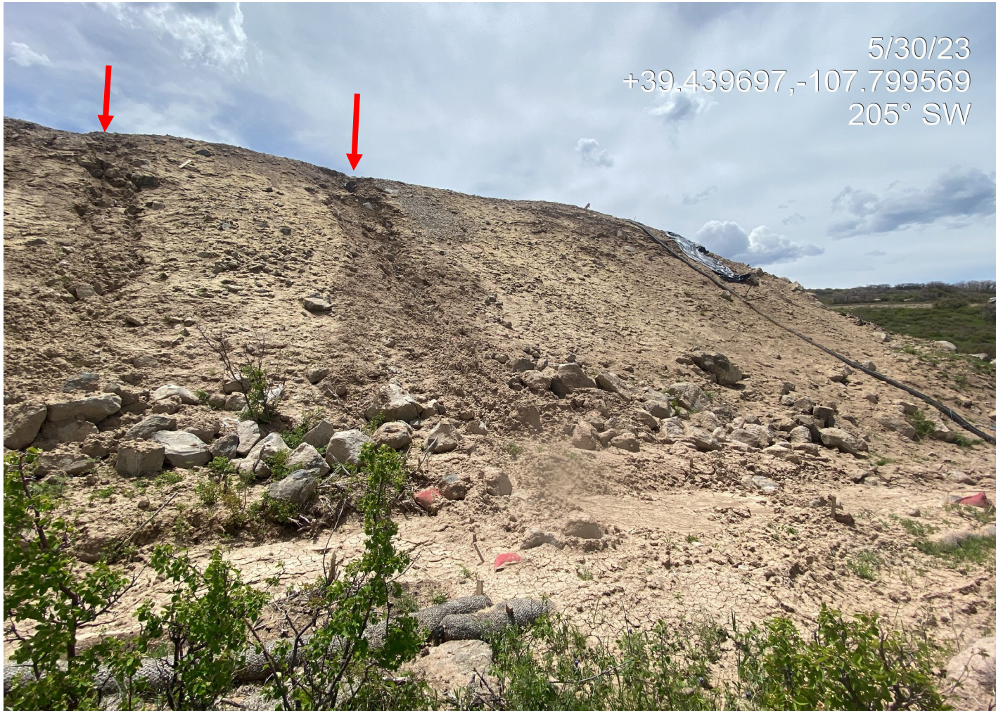
Photo 17. Photo shows the fill slope is unstabilized. Sediment from gully erosion has filled in and overtopped perimeter stormwater BMPs and is being transported offsite.
