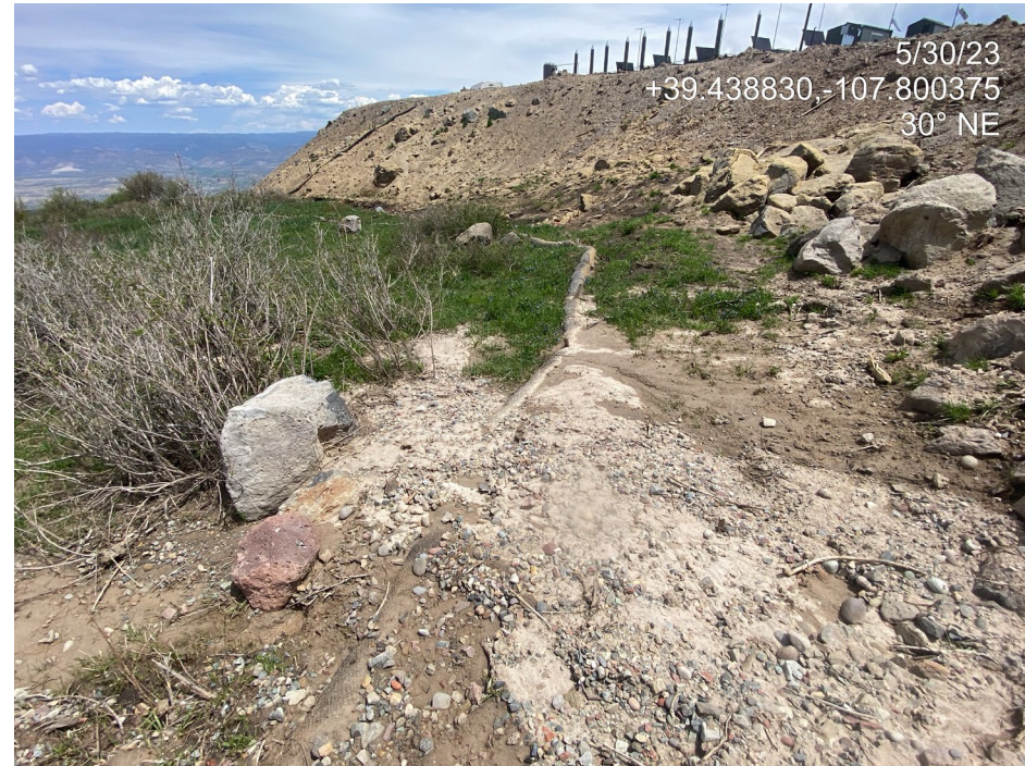
Photo 21. Photos taken from the access road to the west of the location. Stormwater is bypassing a culvert and eroding the road fill (left) and overtopping wattles, and transporting and depositing sediment in undisturbed areas offsite (right).
