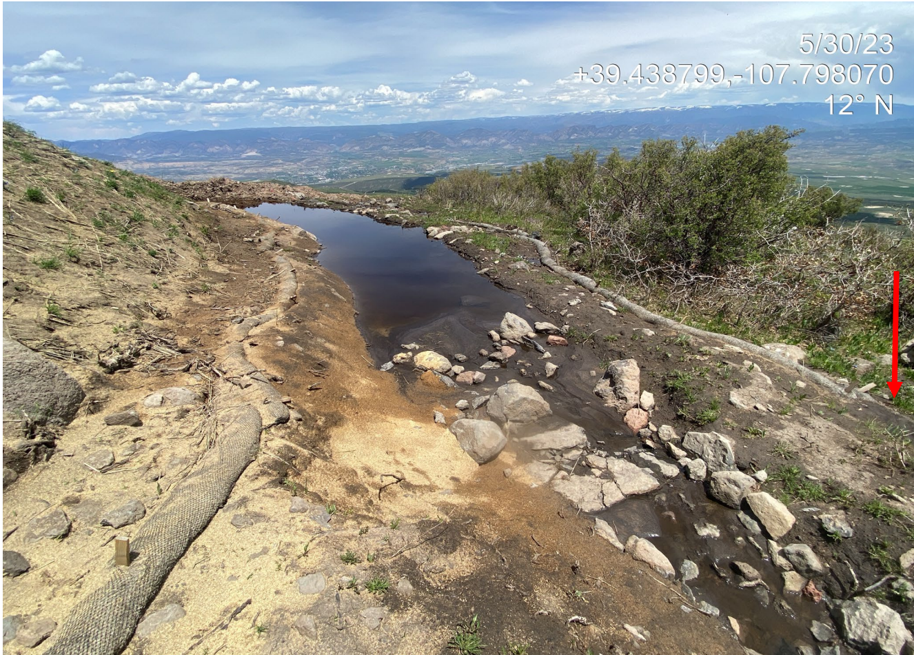
Photo 9. Photo shows a sediment trap at the northeast. The inlet is degraded via scouring, movement/loss of rip-rap and sediment deposition. Sediment laden stormwater is exiting the ditch and inlet before reaching the trap and overtopping a wattle.
