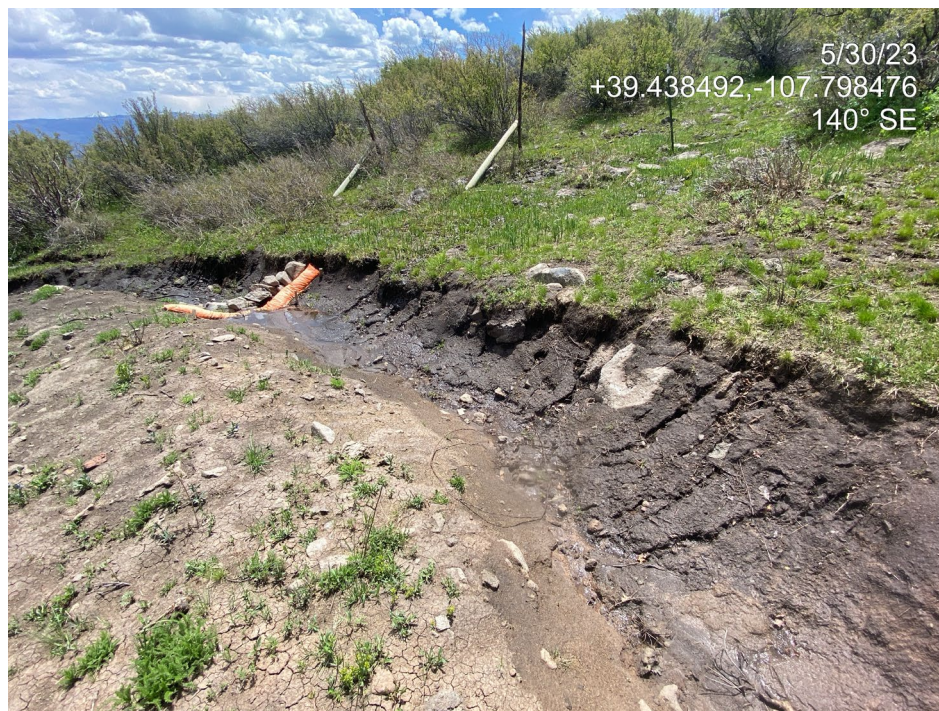
Photo 8. Photos show scouring and rill erosion in the eastern perimeter stormwater ditch resulting in degradation to the BMP and increased sediment loads. Sediment has filled in the check dam.
