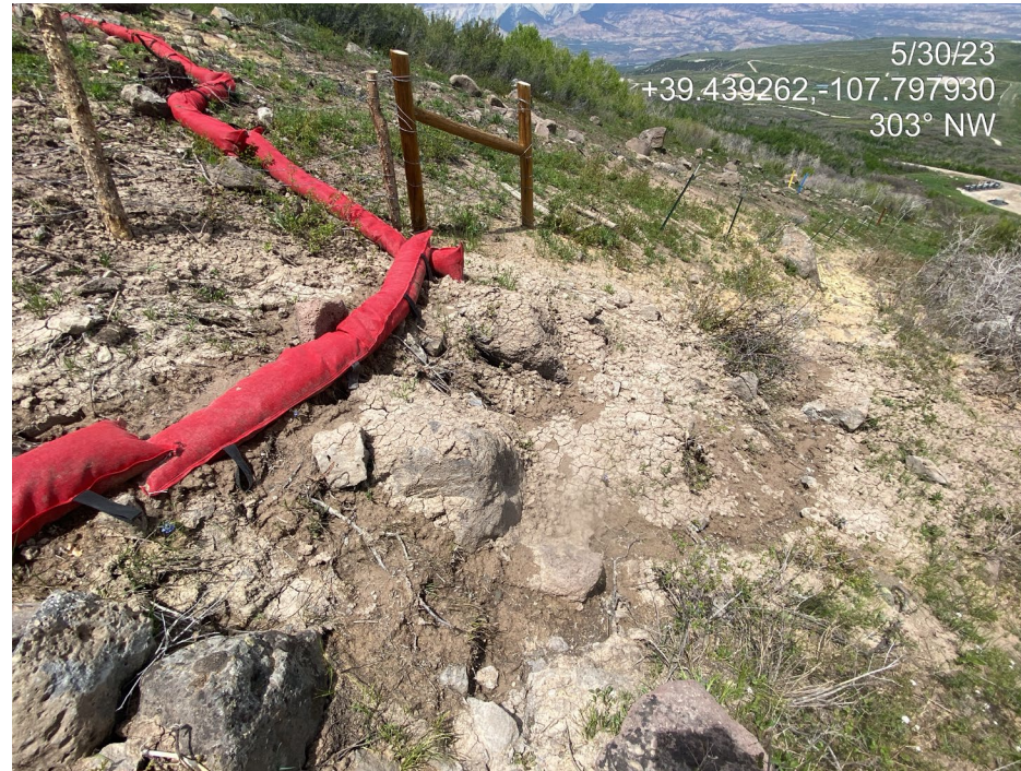
Photo 14. Photos show lack of stabilization BMPs on soils at the east of the location. Sediment is accumulating downslope, offsite.
