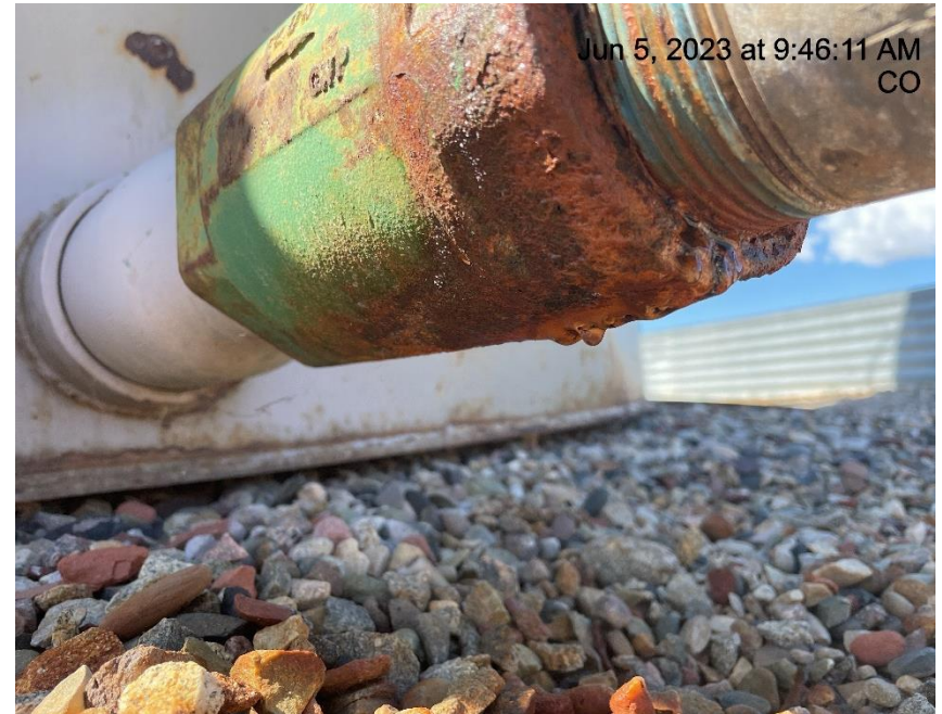
Photo # 9414 Valve on production tank leaking fluid
