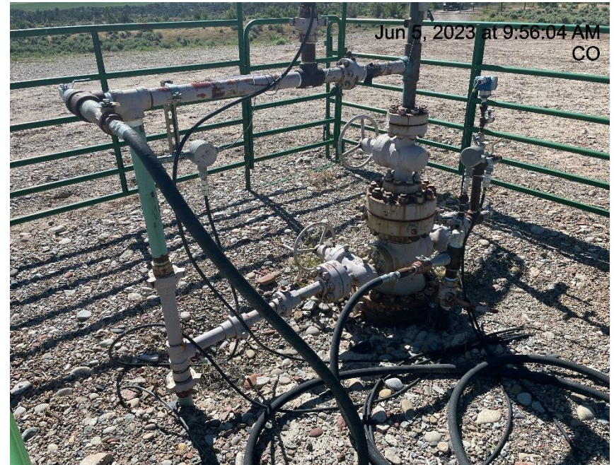
Photo # 9452 Bradenhead hooked into flowline, no check valve observed
