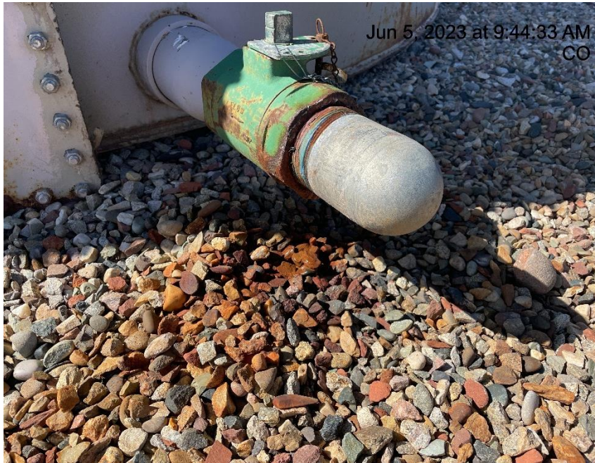
Photo # 9391 Valve on production tank leaking fluid
