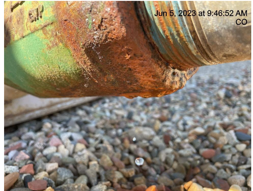
Photo # 9439 Valve on production tank leaking fluid
