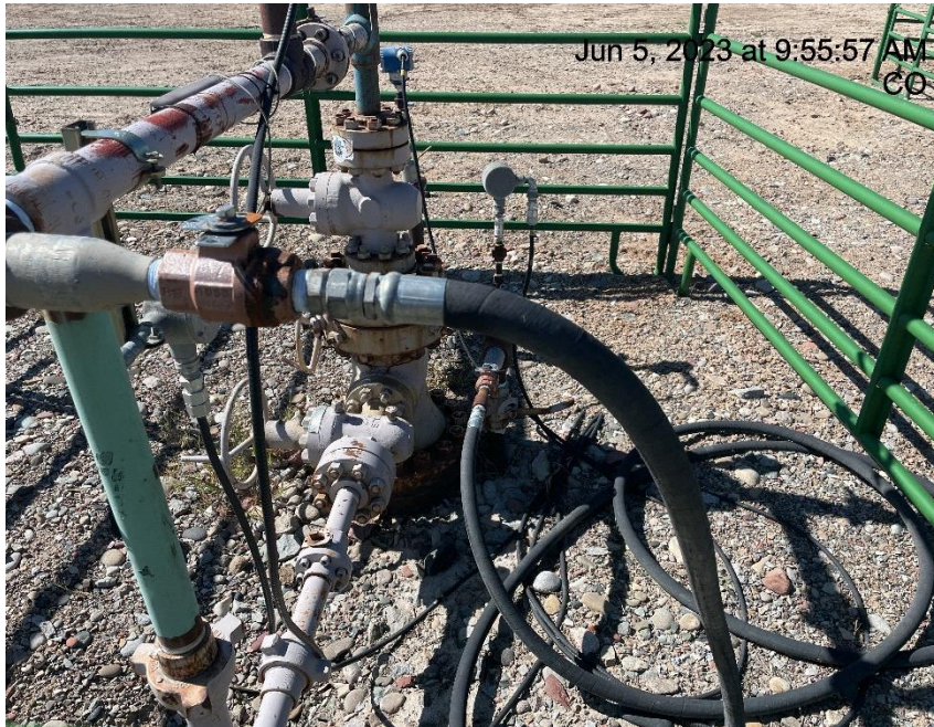
Photo # 9451 Bradenhead hooked into flowline, no check valve observed
