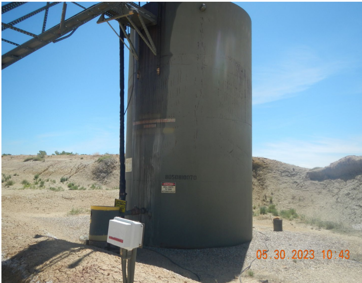
Photo #6 staining on side of tank from overtopping.
