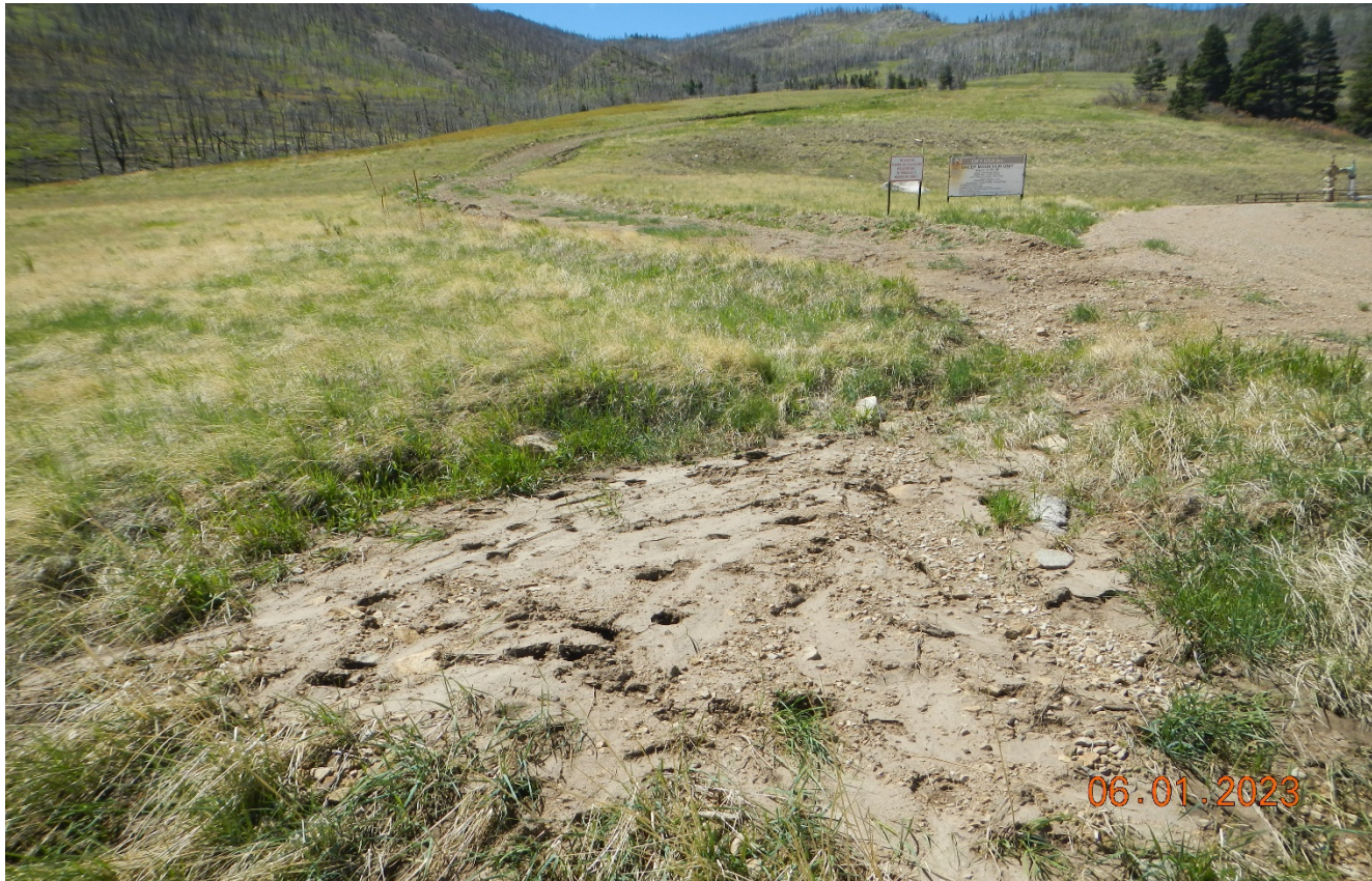
Photo 1. Facing southwest along the access road near the SMU #1-12-B . There is sediment from the road depositing in this area off the road causing additional disturbance. BMP's such as a sediment trap should be installed in this area.
