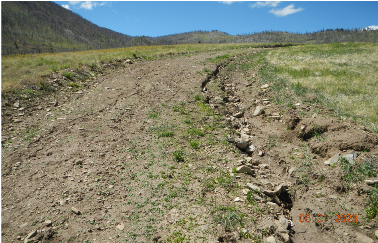
Photo 3. Facing southwest further along the access road. There is erosion occurring along the access road and no BMP's were installed since previous inspection.
