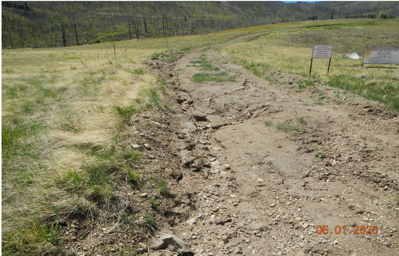
Photo 2. Facing southwest along the access road near the SMU #1-12-B . The is erosion occurring along the access road and no BMP's were installed since previous inspection.
