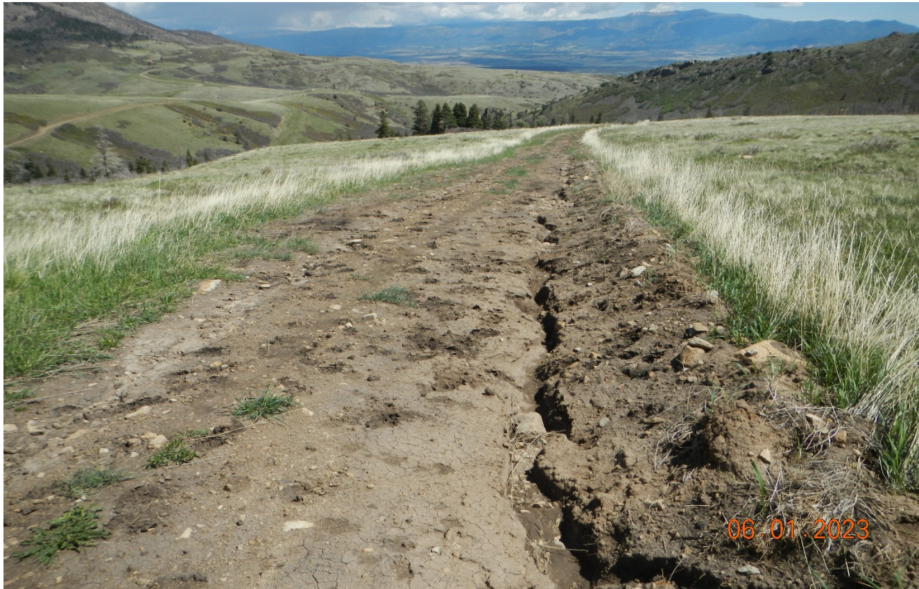
Photo 4. Facing back to the northeast. The road is directing stormwater all the way down the road causing erosion. No BMP's have been installed to direct stormwater off the road and reduce stormwater concentration along the road. Previous corrective action has not been completed.
