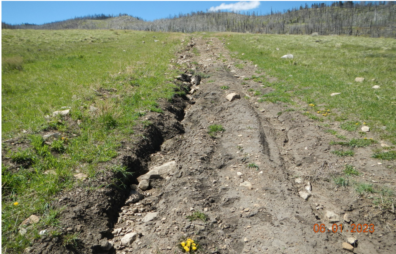
Photo 5. Facing southwest further along the access road. There are areas of erosion occurring which need to be repaired and stabilized. Previous corrective action has not been completed.
