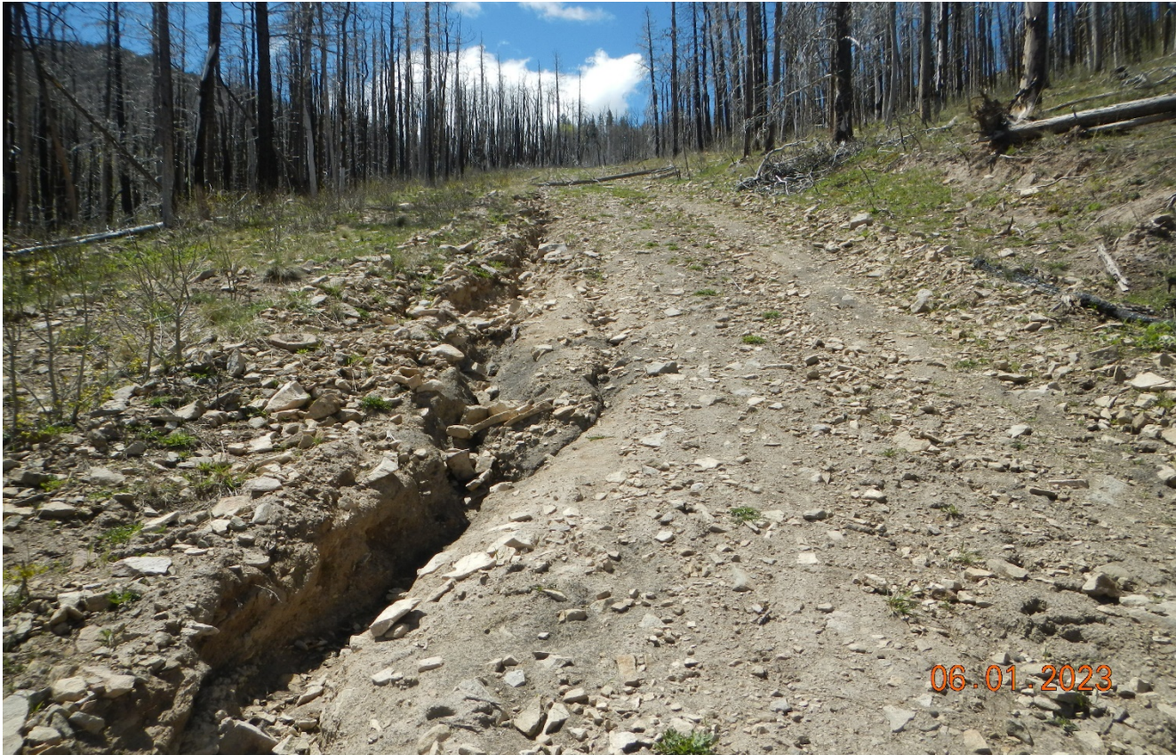
Photo 8. Facing southwest further along the access road. There are areas of erosion occurring which need to be repaired and stabilized. Previous corrective action has not been completed.
