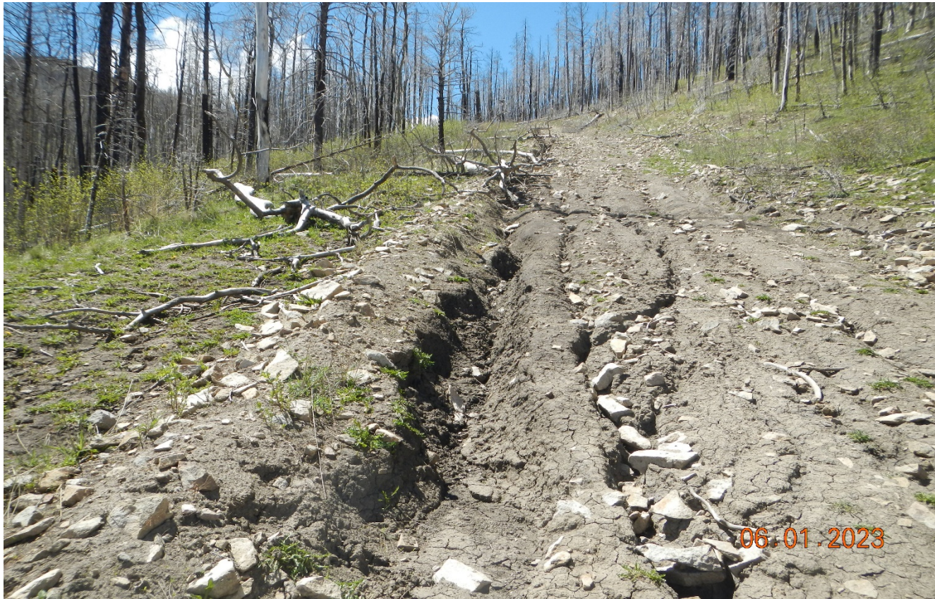
Photo 7. Facing southwest further along the access road. There are areas of erosion occurring which need to be repaired and stabilized. Previous corrective action has not been completed.
