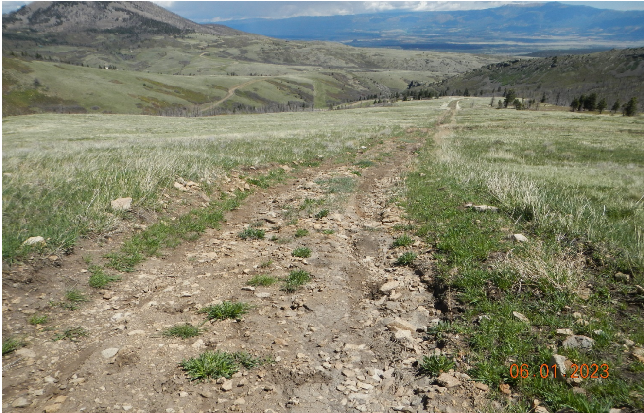
Photo 6. Facing back northeast along the access road. Stormwater is directed all the way down the length of the road with no BMP's to divert and control stormwater. Previous corrective action has not been completed.
