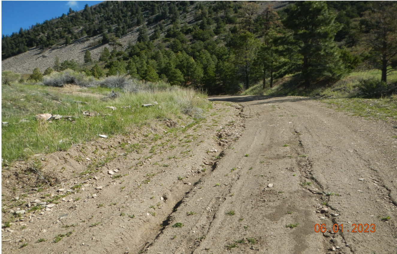
Photo 5. There is erosion occurring on the access road to the location.
