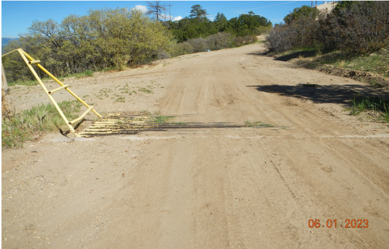
Photo 1. Facing northwest along the access road. This cattle guard has filled in with sediment and is obstructing stormwater flow along the right side of the road.
