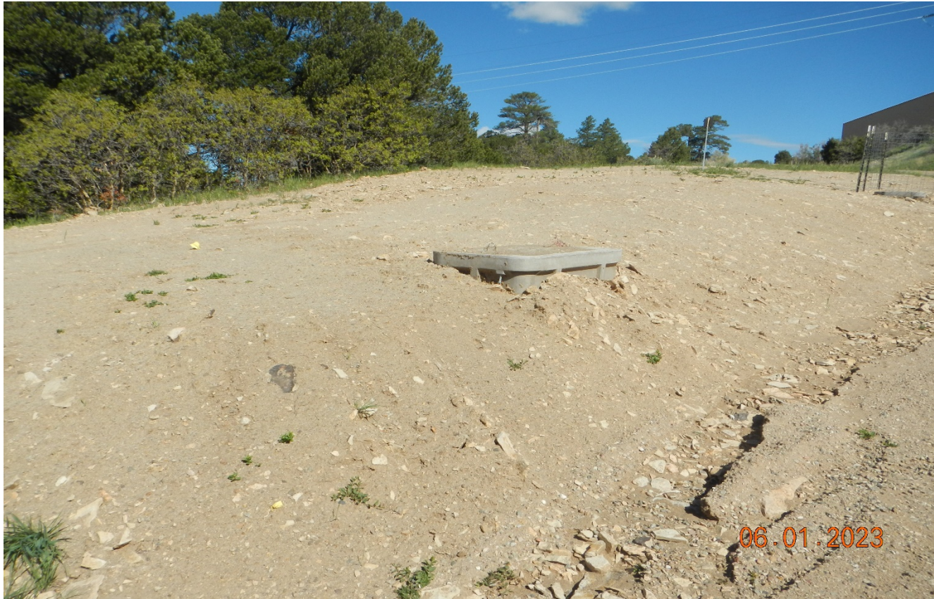
Photo 4. The flowline disturbance area was reseeded last year but vegetation does not appear to be establishing.
