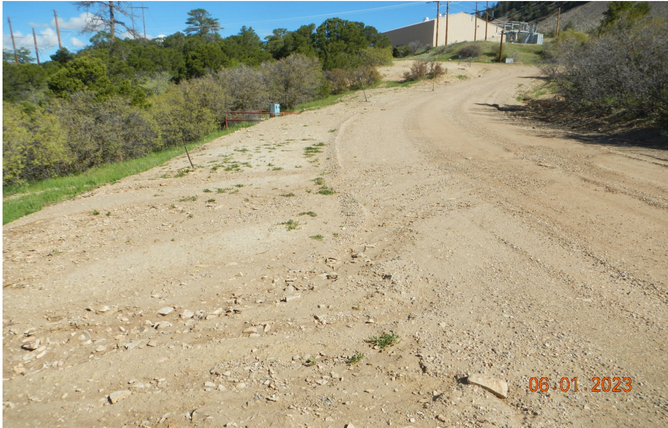
Photo 2. Stormwater is not being properly diverted and is causing erosion across the road transporting sediment offsite shown in the next photo.
