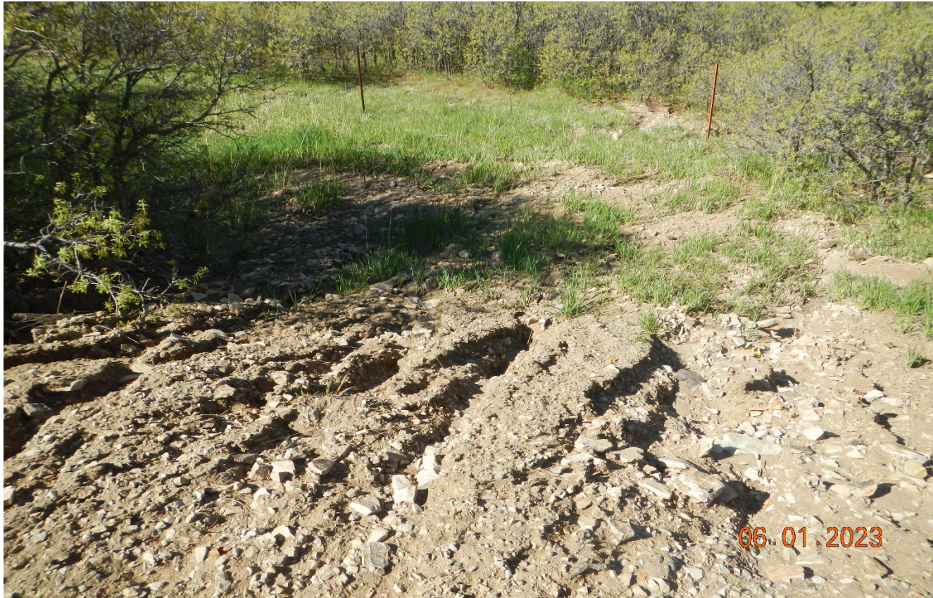
Photo 3. There is erosion of the road side occurring in this same area of previous photo.
