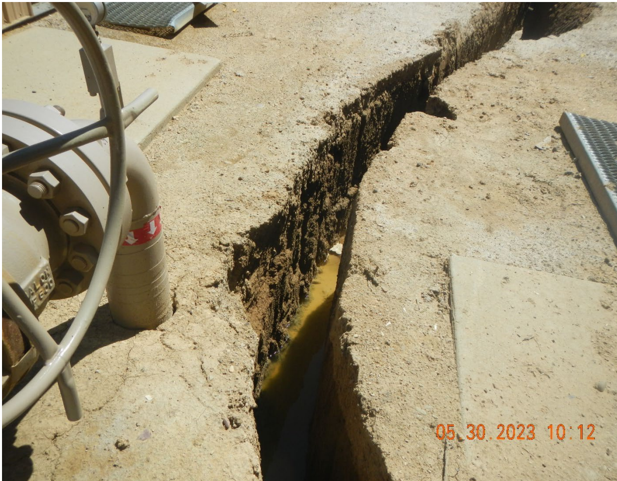
Photo #3 hydro excavation to expose trench for new line.
