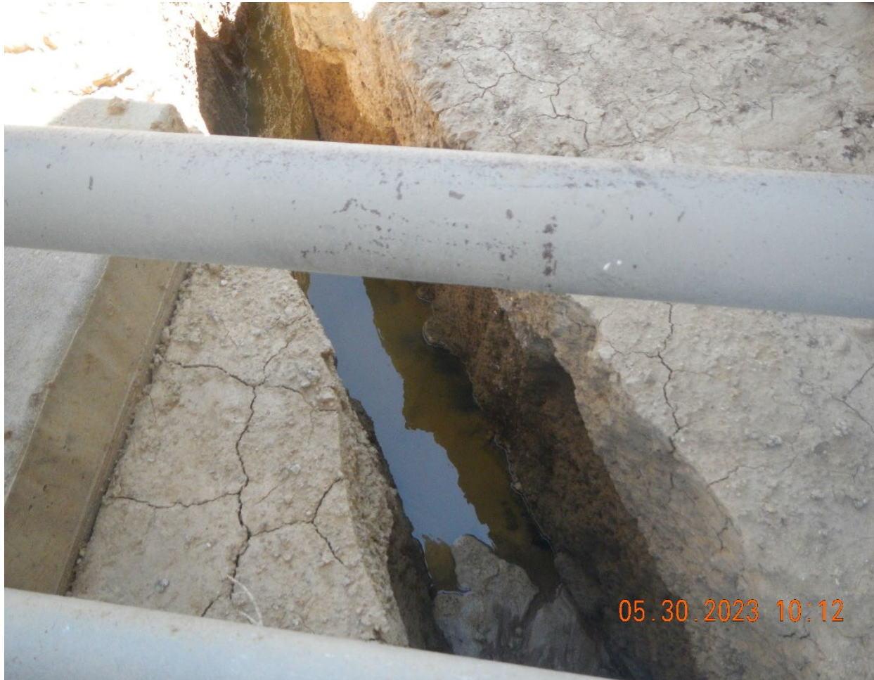
Photo #2 hydro excavation to expose trench for new line.
