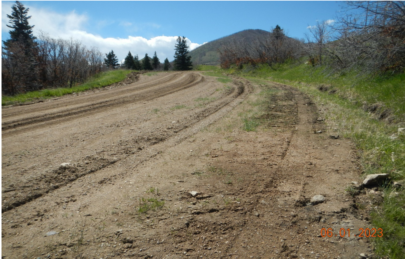
Photo 3. Facing southeast ascending the hill toward the location. The road has been widened along this area which will create more stormwater impact. Disturbance area of the road needs to be minimized.
