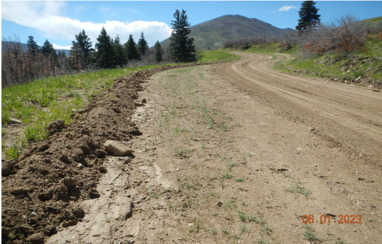
Photo 1. Facing southeast ascending the hill toward the location. Grading has pushed out material into a berm which is creating more of a disturbance and not allowing stormwater to be diverted off the road. There is a long stretch of the road where stormwater will be directed down the road which will cause erosion.
