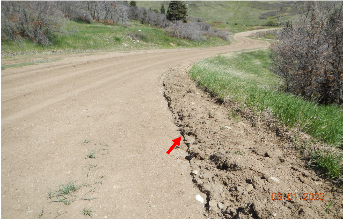
Photo 2. Facing southeast ascending the hill toward the location. Stormwater is not diverted off the road and the an erosion channel is beginning to develop.
