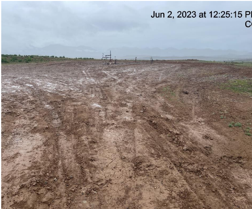
Photo # 9278 Lack of stabilization/compaction /insufficient BMP's on location
