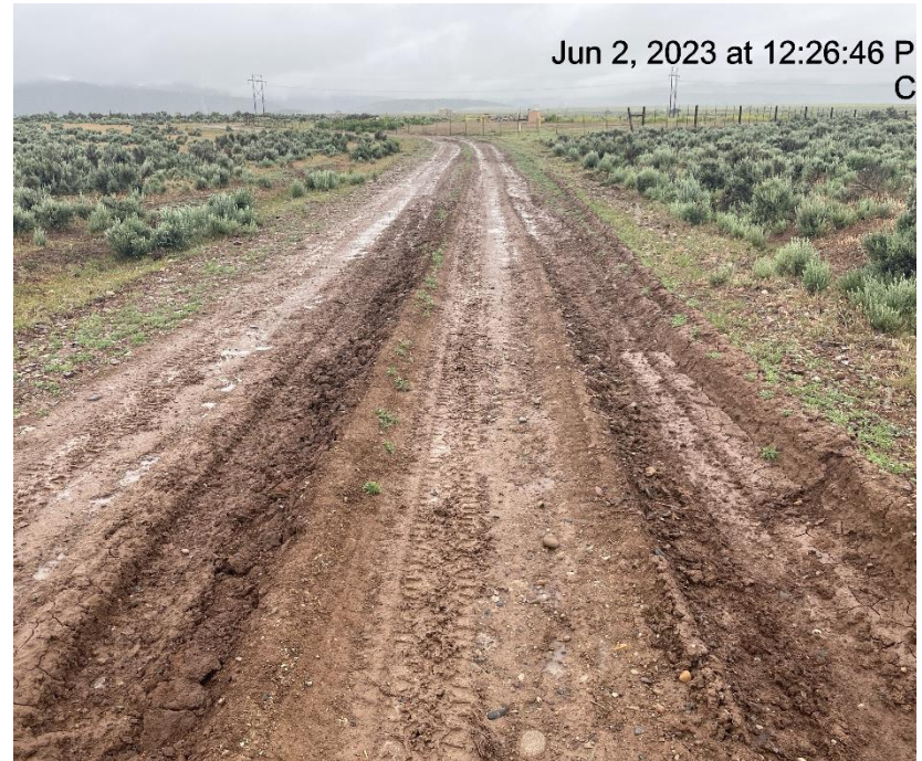
Photo # 9281 Lack of stabilization/compaction /insufficient BMP's on lease road
