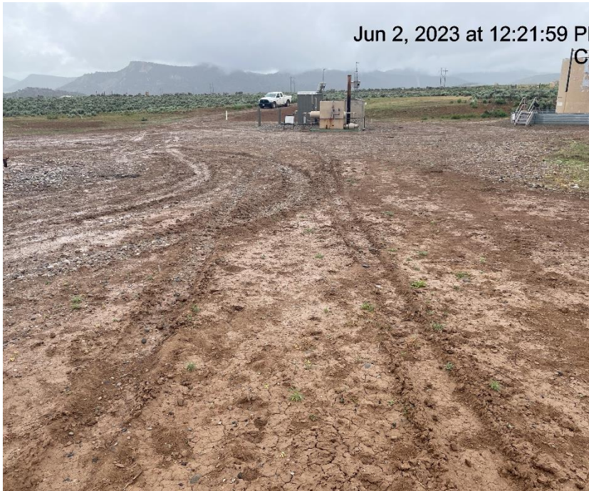
Photo # 9271 Lack of stabilization/compaction /insufficient BMP's on location
