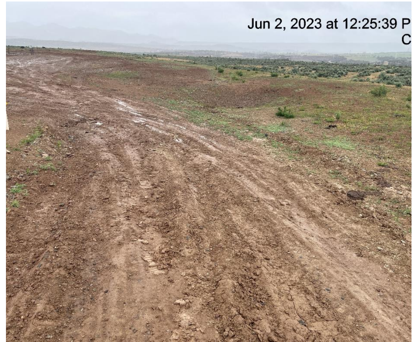
Photo # 9279 Lack of stabilization/compaction /insufficient BMP's on location & lease road
