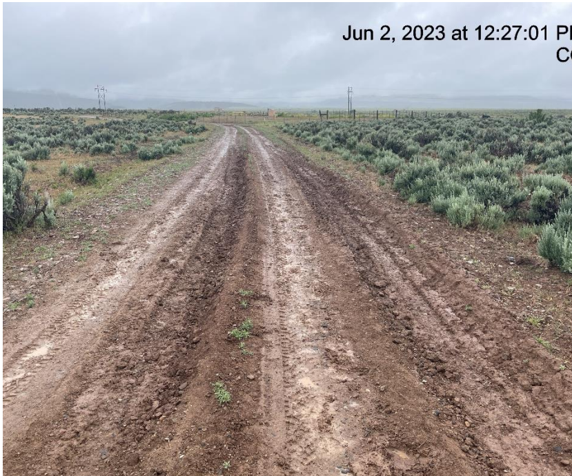
Photo # 9282 Lack of stabilization/compaction /insufficient BMP's on lease road
