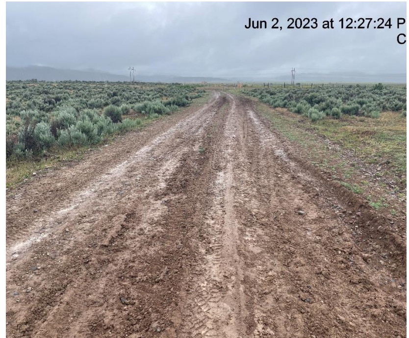
Photo # 9283 Lack of stabilization/compaction /insufficient BMP's on lease road
