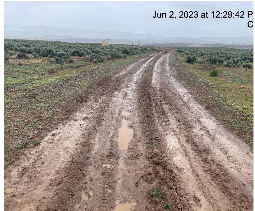
Photo # 9286 Lack of stabilization/compaction /insufficient BMP's on lease road
