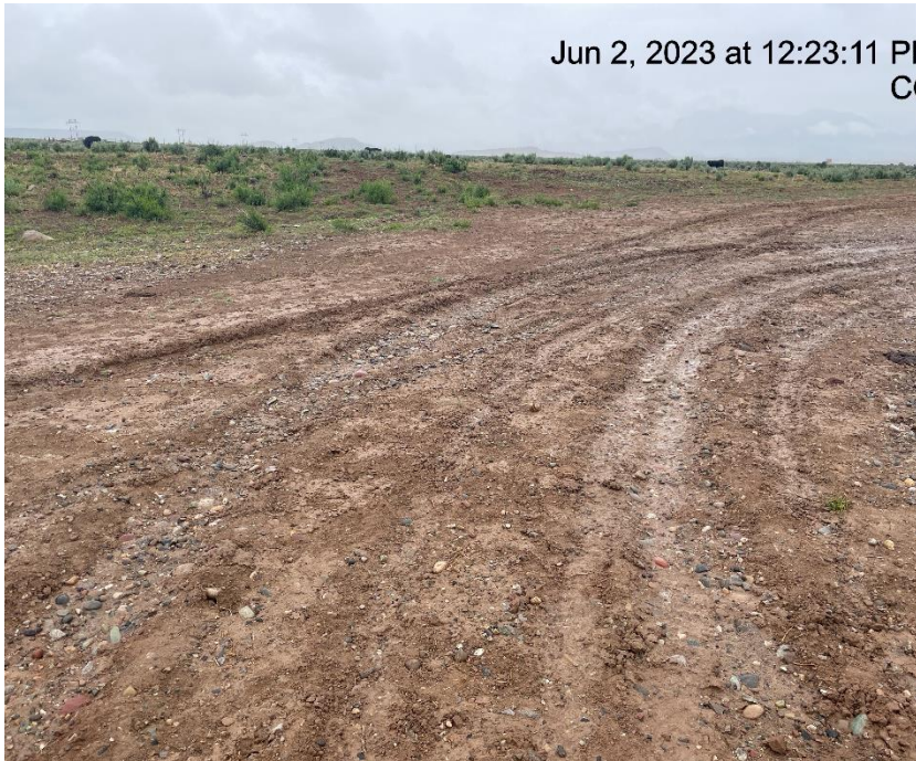
Photo # 9275 Lack of stabilization/compaction /insufficient BMP's on location
