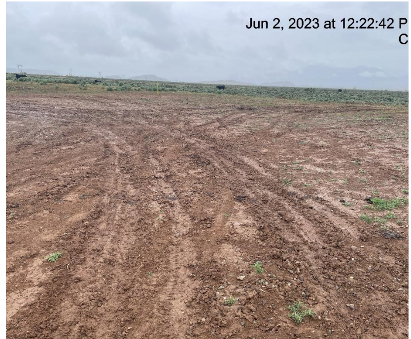
Photo # 9274 Lack of stabilization/compaction /insufficient BMP's on location
