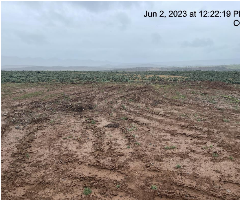
Photo # 9273 Lack of stabilization/compaction /insufficient BMP's on location
