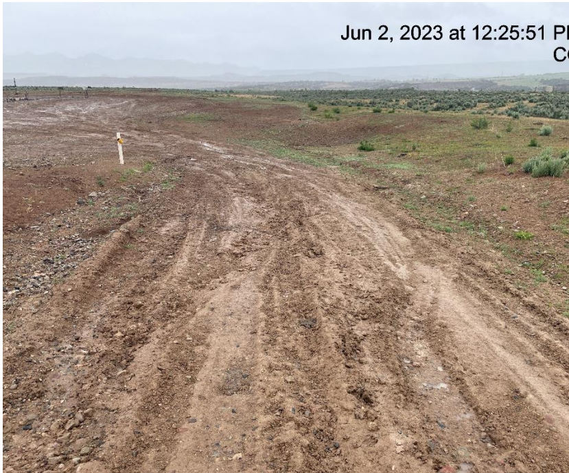
Photo # 9280 Lack of stabilization/compaction /insufficient BMP's on lease road
