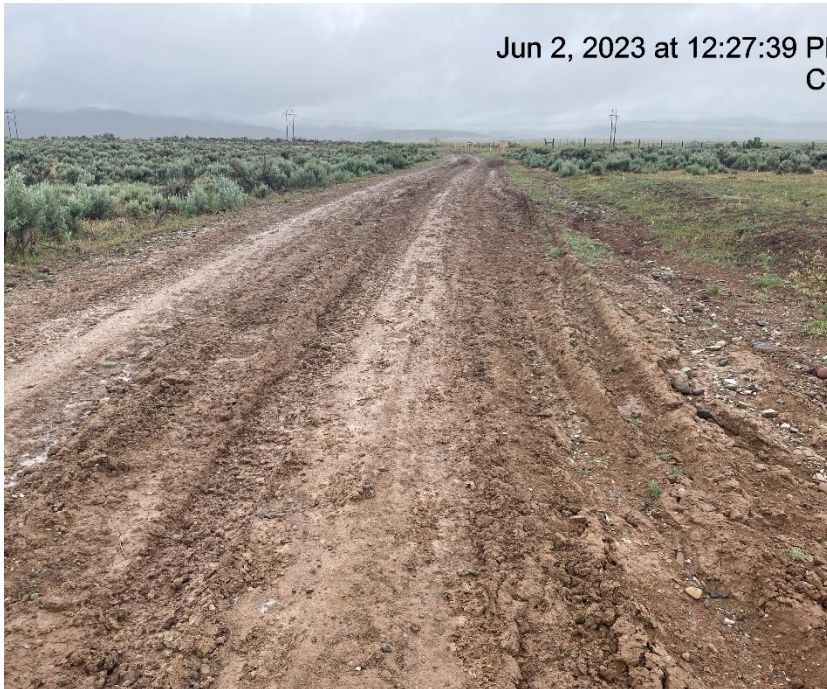
Photo # 9284 Lack of stabilization/compaction /insufficient BMP's on lease road
