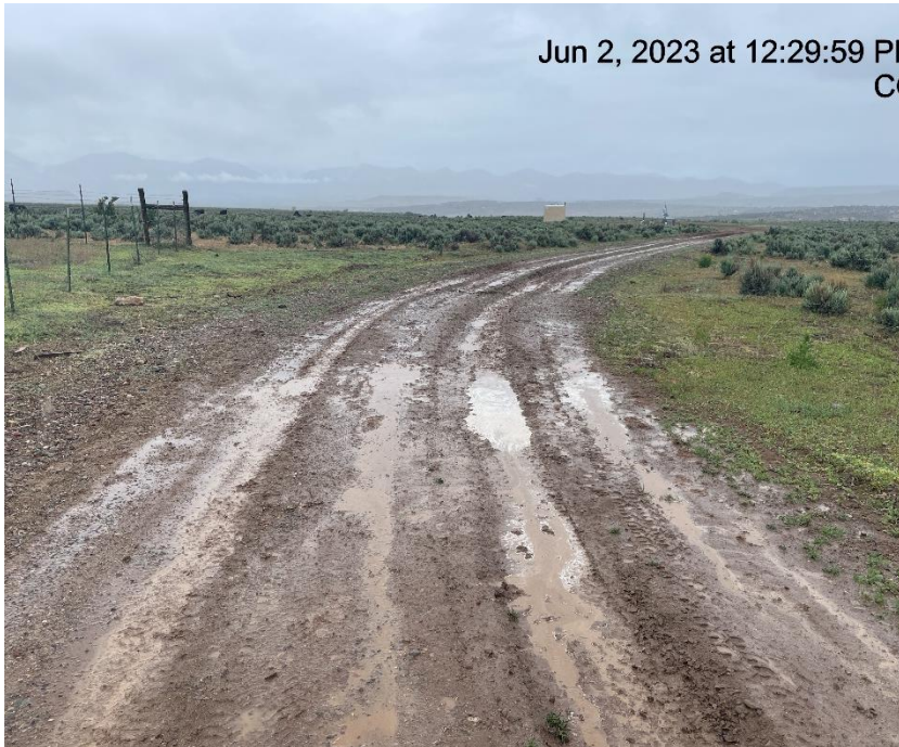
Photo # 9287 Lack of stabilization/compaction /insufficient BMP's on lease road
