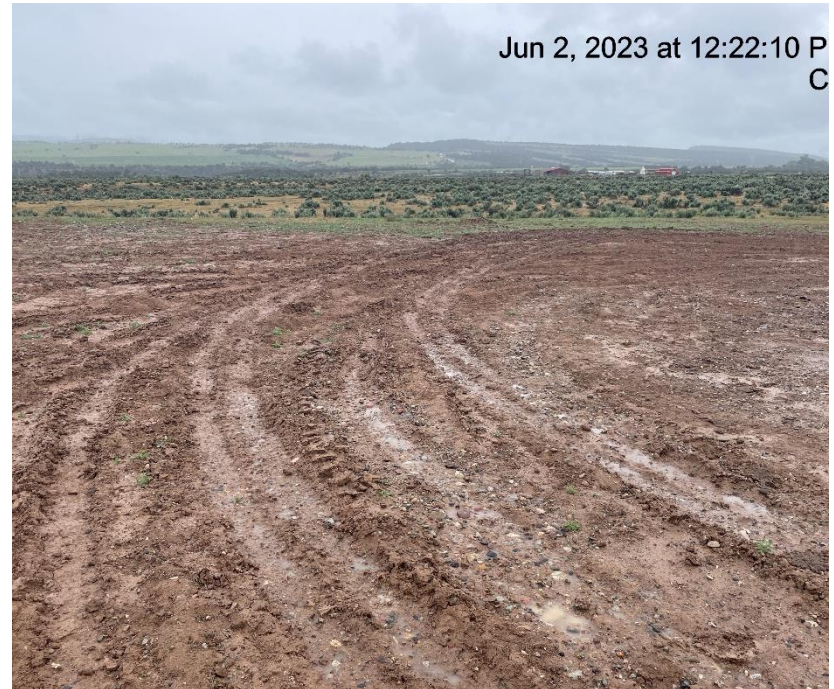
Photo # 9272 Lack of stabilization/compaction /insufficient BMP's on location
