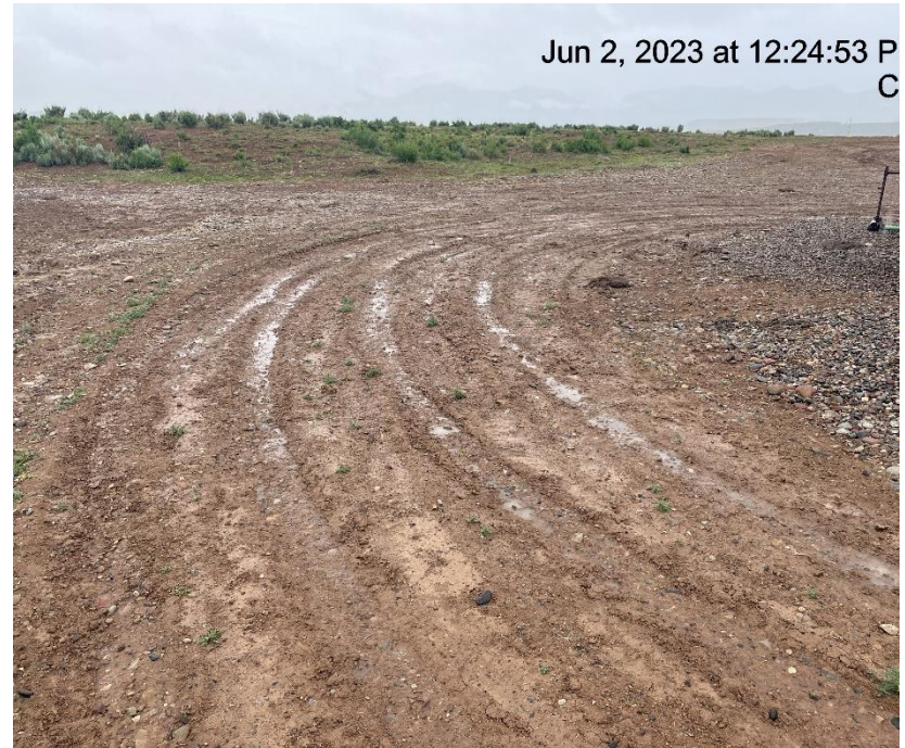
Photo # 9277 Lack of stabilization/compaction /insufficient BMP's on location
