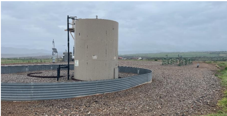
South West corner of location.
