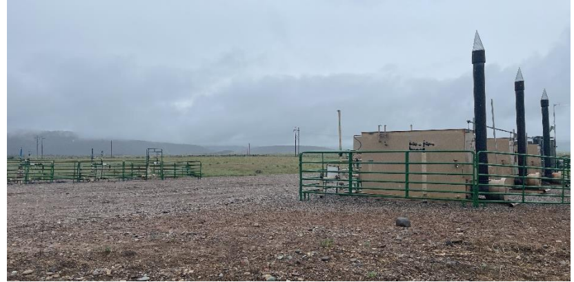
North East corner of location.
