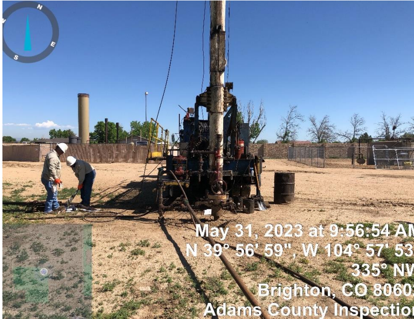
Photo#1 Wellhead/Crew hooking up Swab Rig
