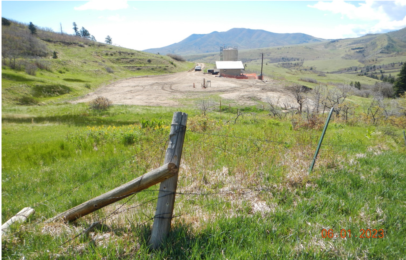
Photo 9. Facing southeast further away from the location. There is a degraded perimeter fence that needs to be maintained.
