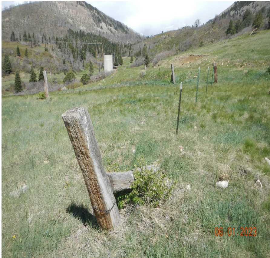
Photo 13. Observed along the access road were several dilapidated snow fences which need to be removed or repaired.
