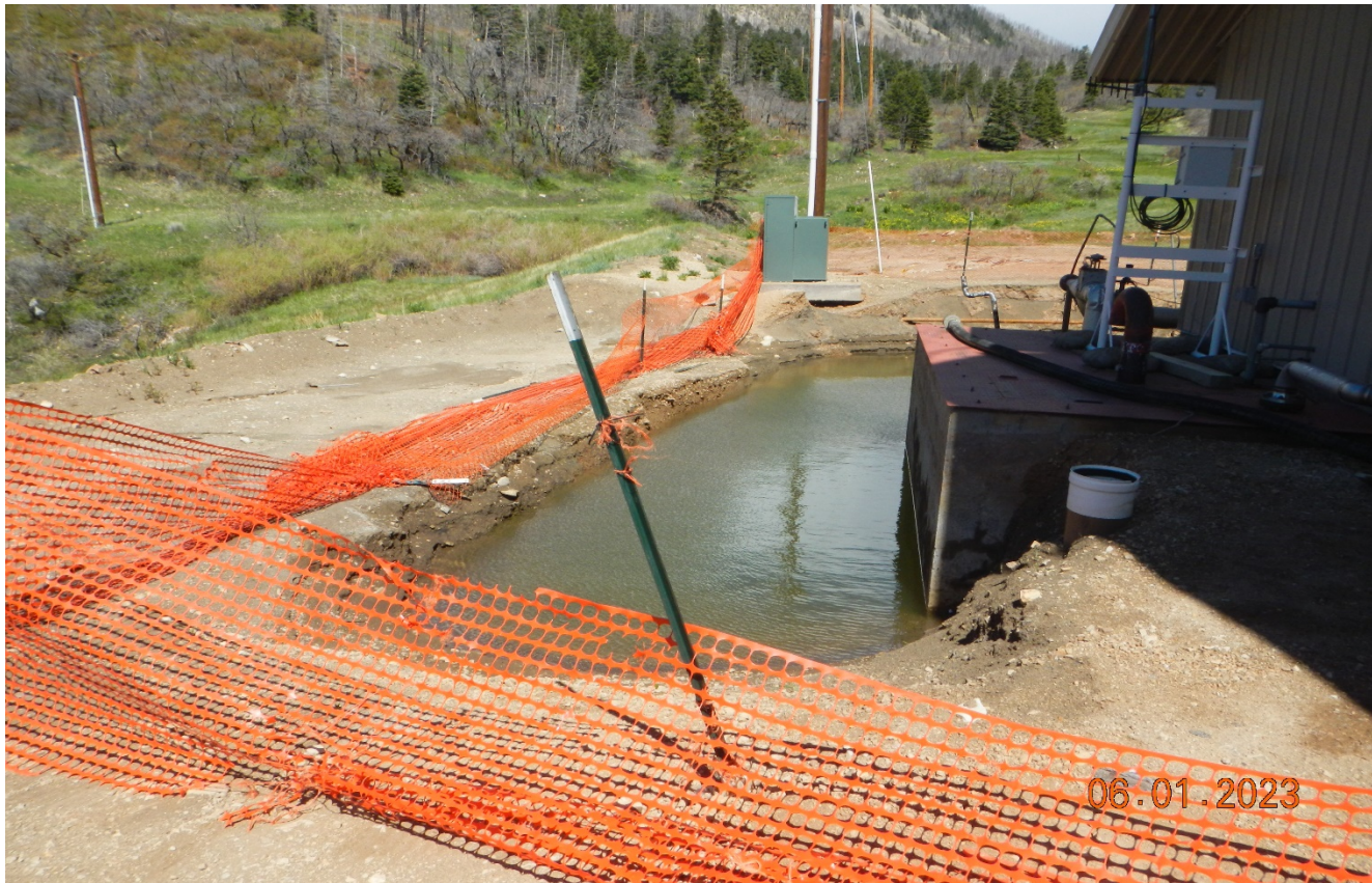
Photo 4. Facing northwest at the location. The remediation area where tank was located remains open and the safety fence is in disrepair. Previous corrective action was not completed.
