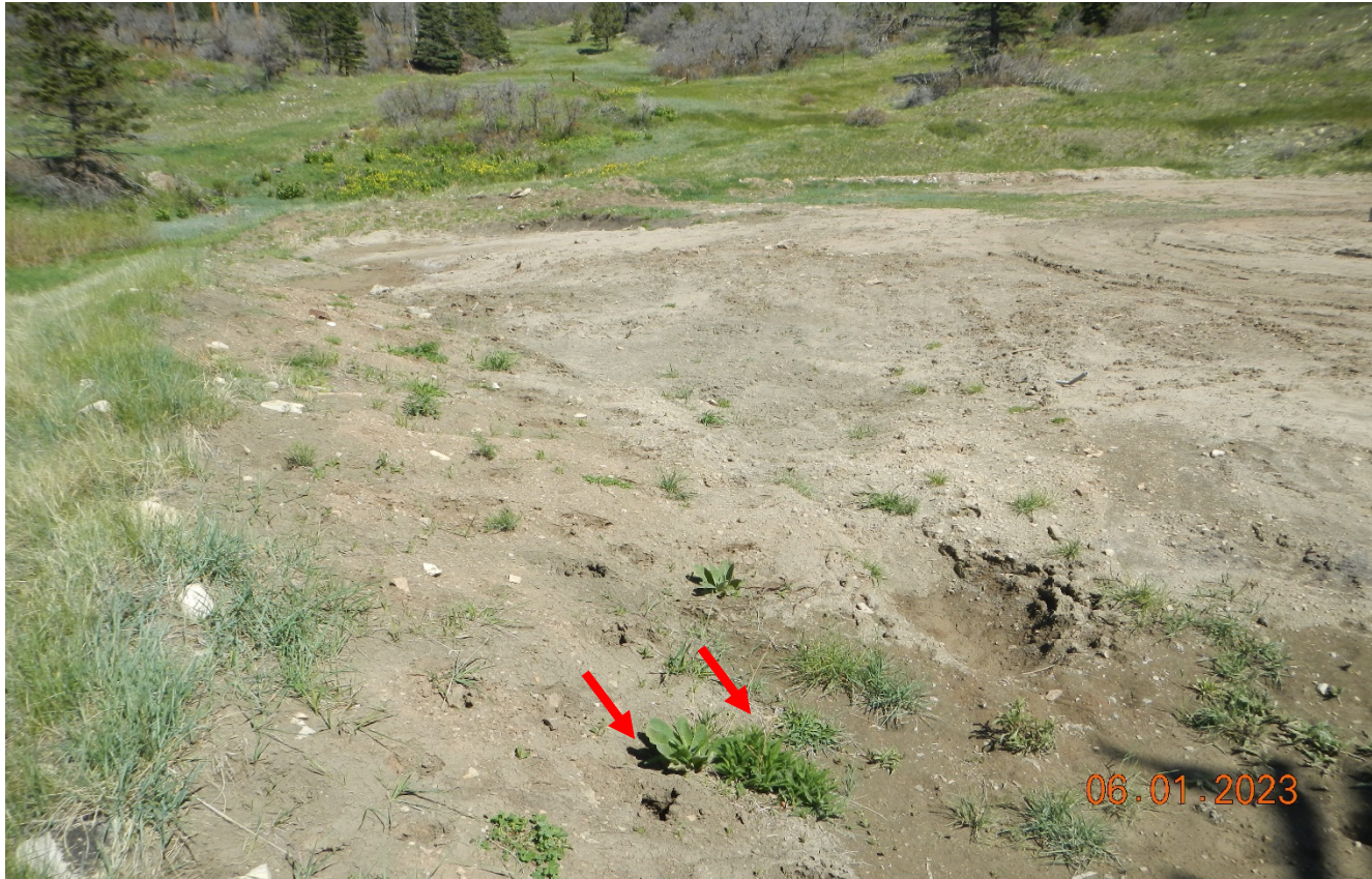
Photo 6. Facing northwest toward the excavated area which has been backfilled. There are noxious weeds shown at red arrow and the disturbed soils need to be recontoured and reclaimed.
