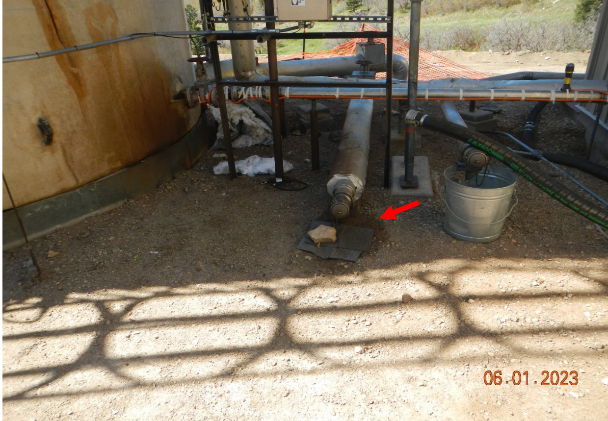
Photo 2. There is still stained soil at the pipe outlet. Previous corrective action was not completed. There is also insulation debris that needs to be removed.
