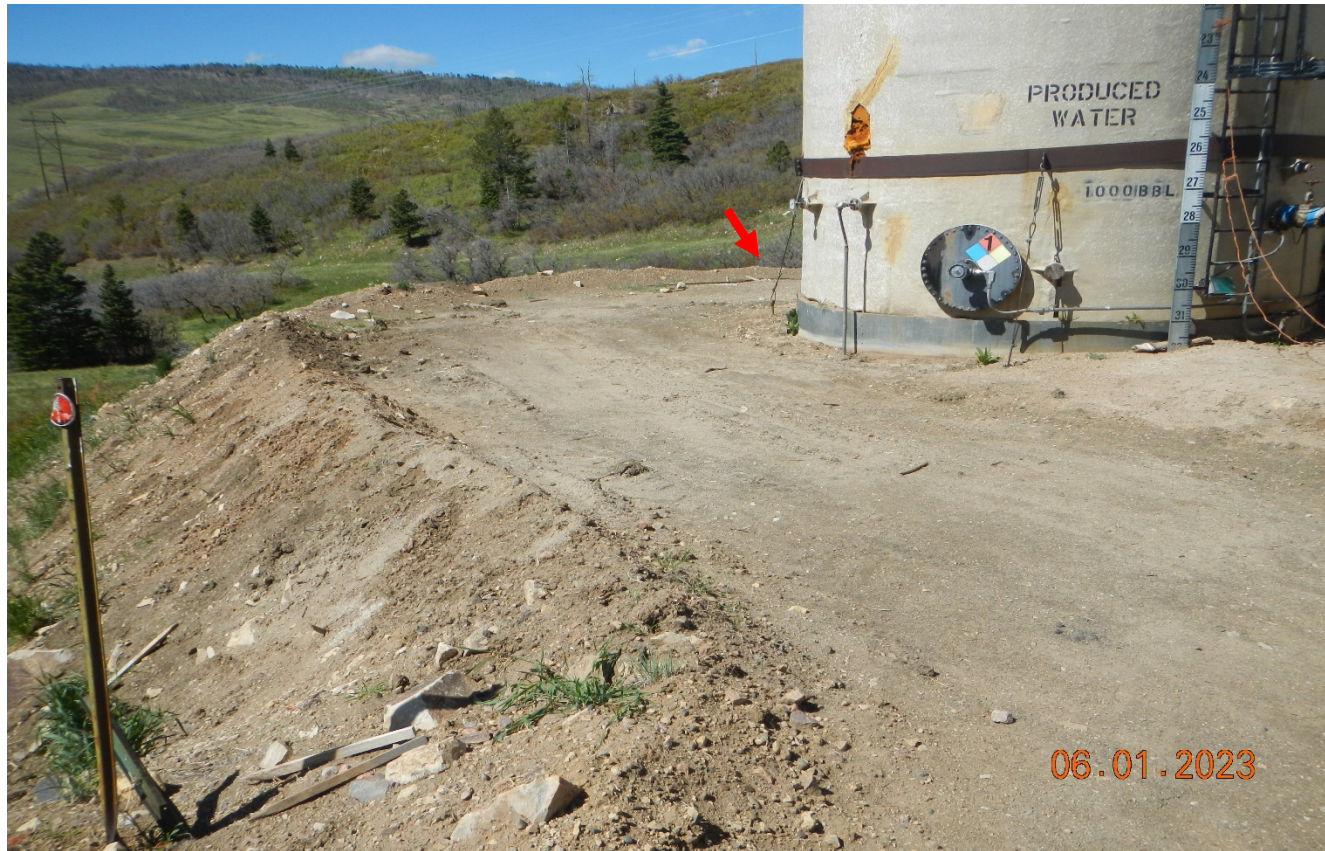
Photo 3. Facing toward the produced water tank. The secondary berm around the tank is insufficient to contain a spill. Red arrow points to small berm which could easily be overtopped by a leak. Previous corrective action was not completed.
