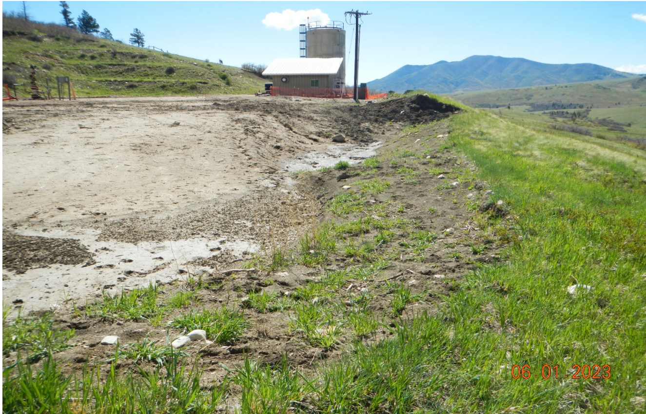
Photo 7. Facing southeast at the down gradient portion of the location. The degraded perimeter wattles were removed however, no new BMP's were installed and there is a creek approximately 10ft' from the edge of the location.
