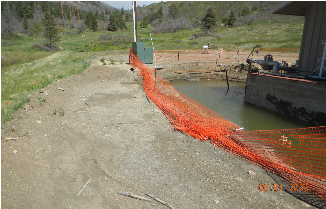
Photo 5. Facing where tank was located which remains an open excavation due to active remediation. Stormwater has filled in the open excavation. Safety fence is in disrepair. Previous corrective action was not completed.
