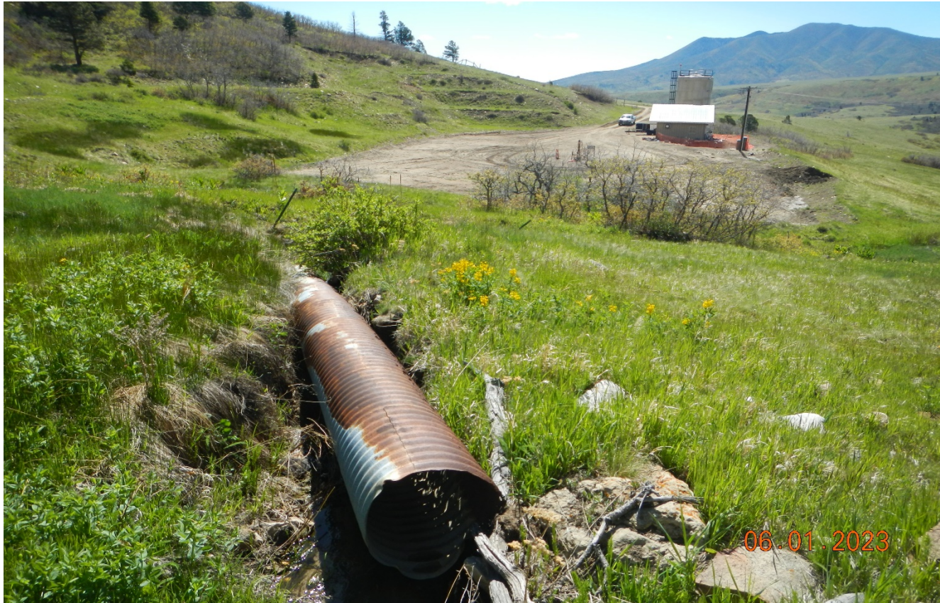
Photo 10. Standing approximately 125' northwest of the location along the flowline area is an eroded out culvert where the creek flows. The culvert needs repaired or removed.
