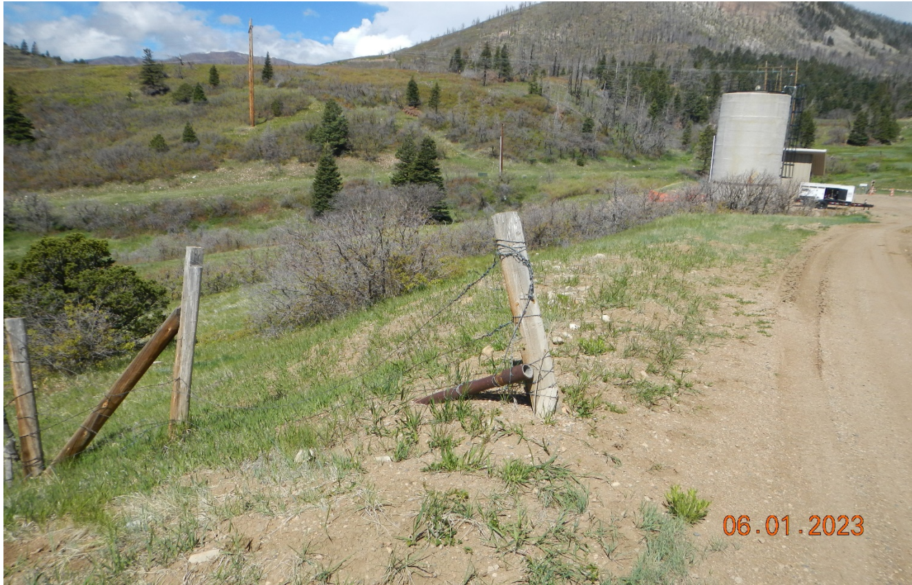
Photo 11. Standing at the east side of the location. The perimeter fence around the location is not maintained and would be beneficial to prevent livestock entry.
