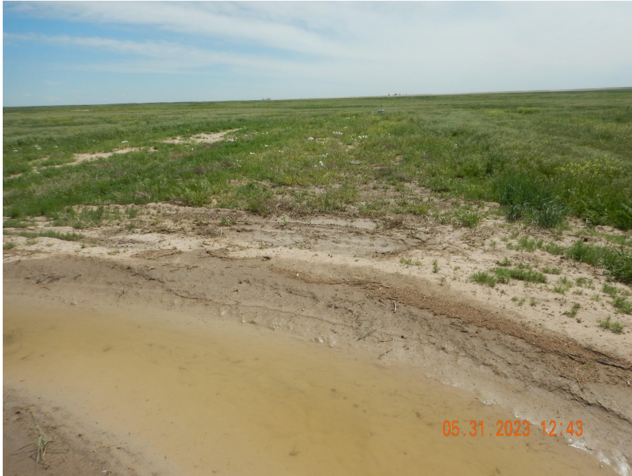
Photo 3. Photo taken from the southwestern perimeter of location, facing South. Photo illustrates sediment laden stormwater has discharged off location. The perimeter ditch and berm BMP is not sufficient.
