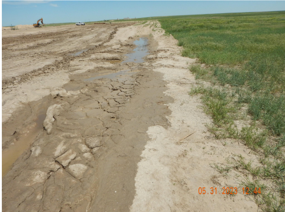
Photo 2. Photo taken from the southwestern perimeter of location, facing East. Photo illustrates vehicle traffic has driven over the perimeter ditch and berm BMP, which was the likely result of sediment laden stormwater discharging off location.
