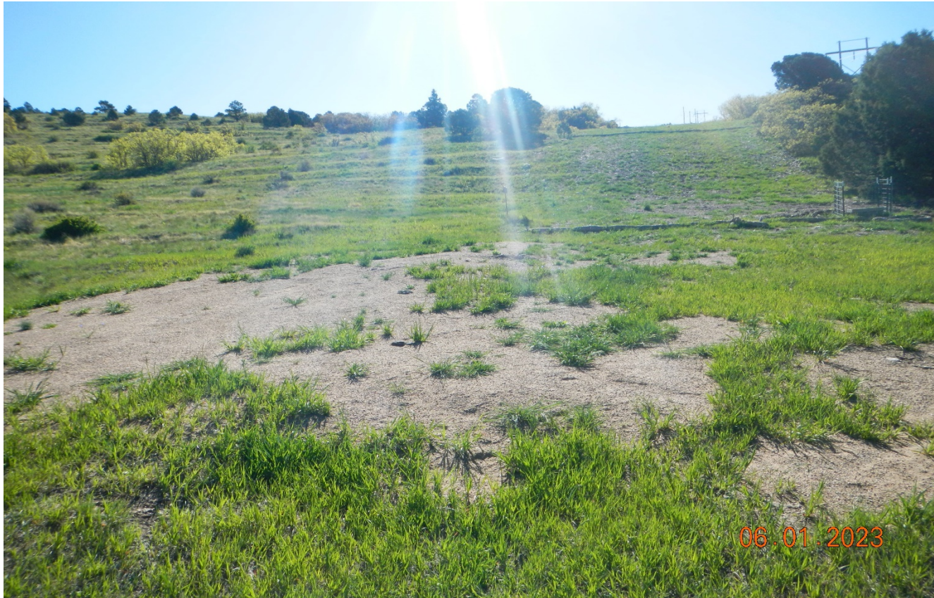
Photo 1. Just west wellsite along the flowline where there was recent disturbance and reclamation. This area has not established vegetation and there is still backfill gravel that remains. This area needs additional reclamation and gravel removal. Lat/Long: 37.6997, -105.20816.
