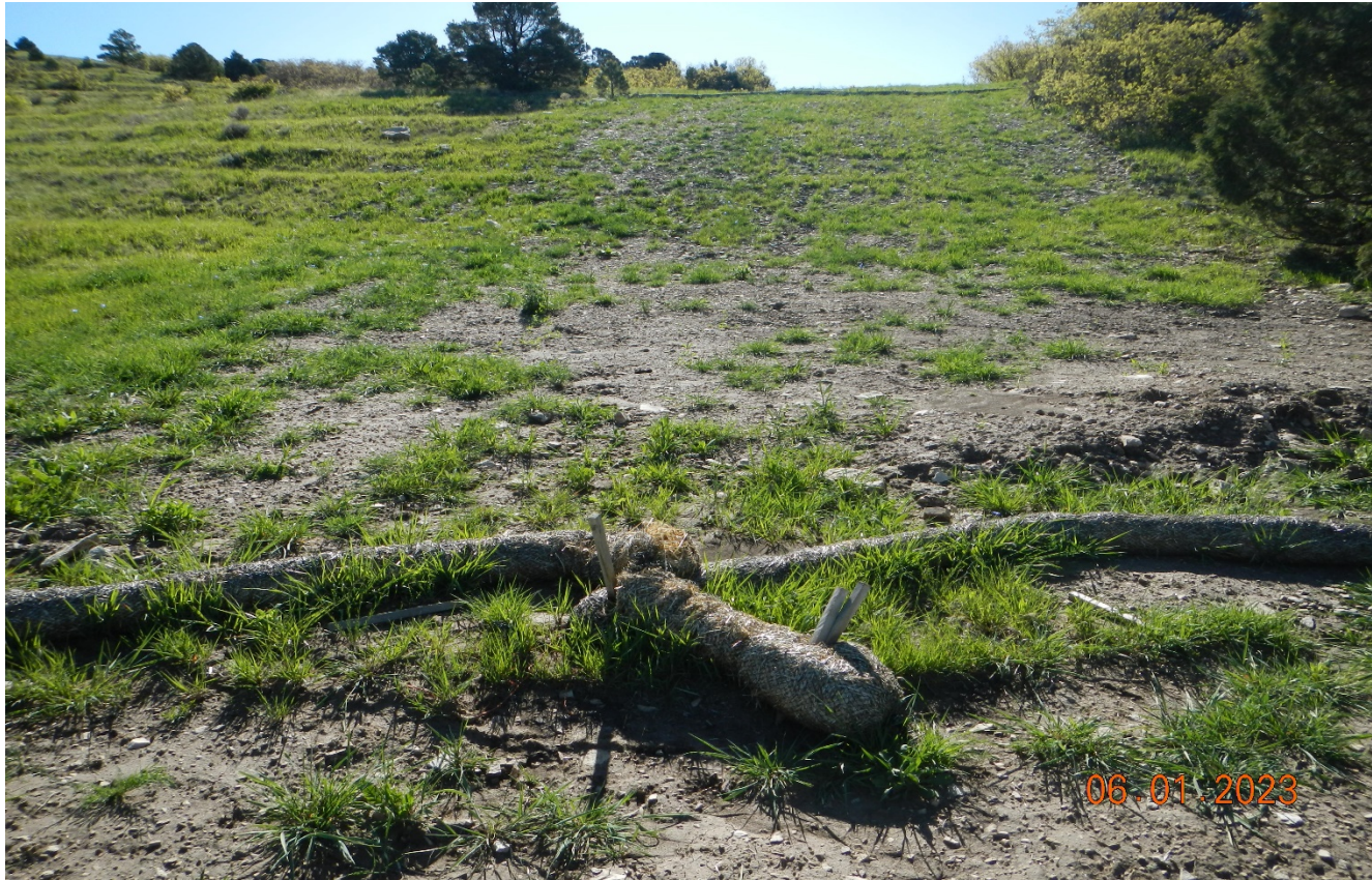
Photo 2. Facing east along the flowline. There is a displaced wattle that needs to be repaired or removed. Lat/Long:37.6997,-105.20816.
