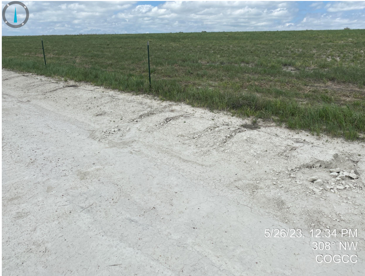
Photo 5. North side of production areas. During this inspection, Staff observed that northern portions of the production area are experiencing rill erosion. Repair/maintenance of stormwater BMPs should be implemented to stabilize the areas experiencing erosion.
