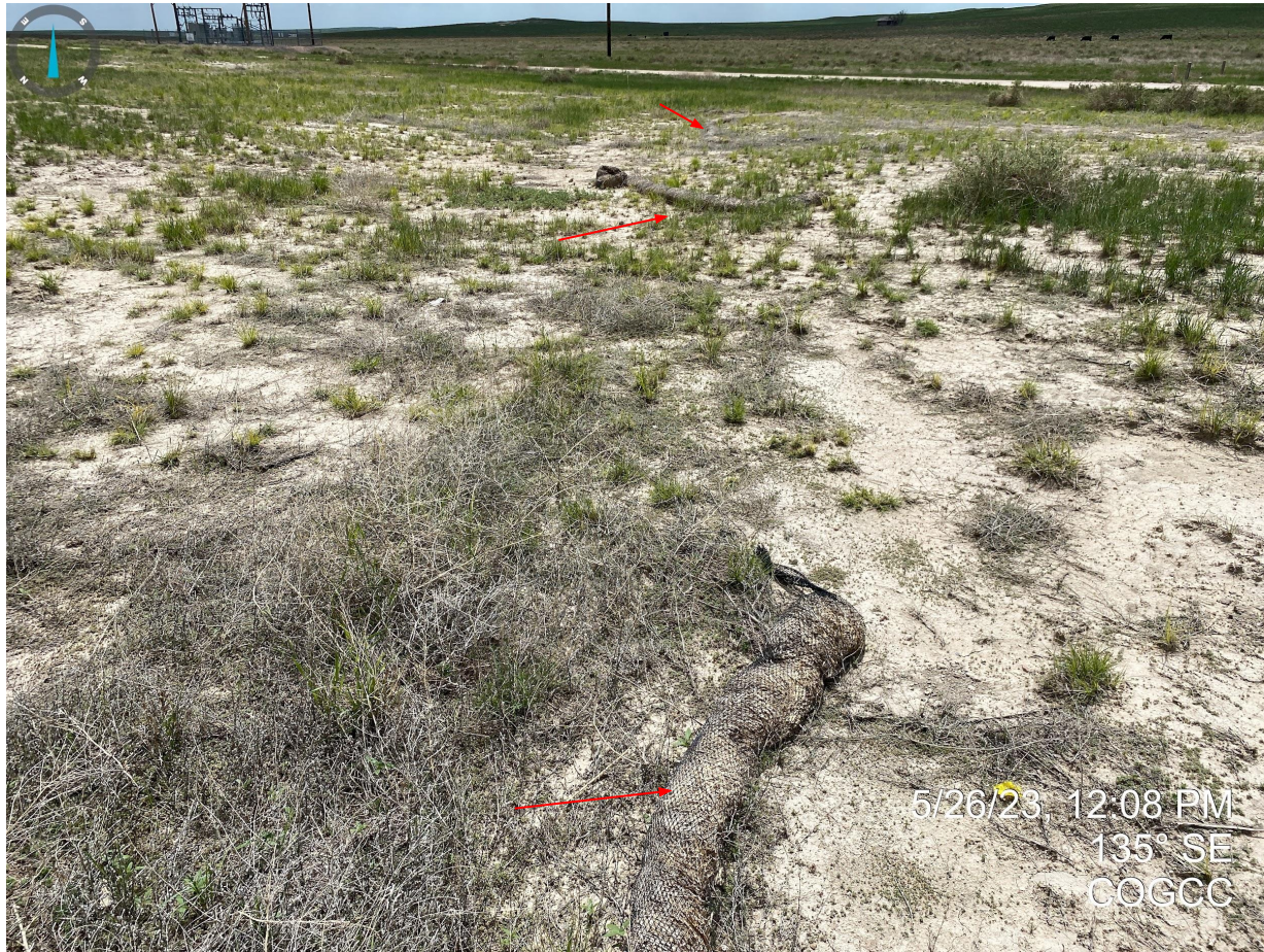
Photo 2. Southern portion of location. Degraded straw wattles are now considered debris and will need to be removed.
