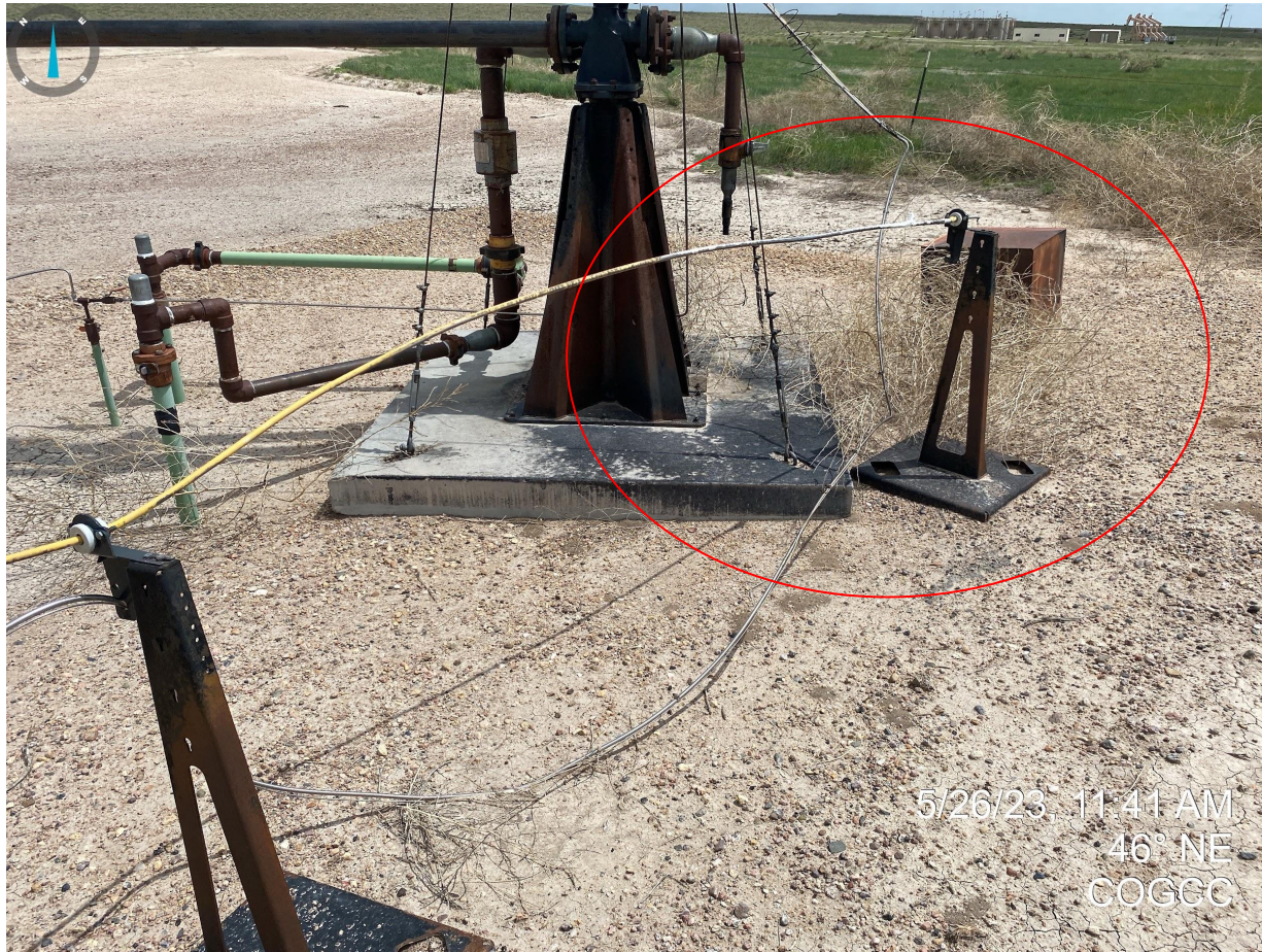
Photo 1. Tumbleweed accumulation around flare will need to be removed as they present a fire hazard.
