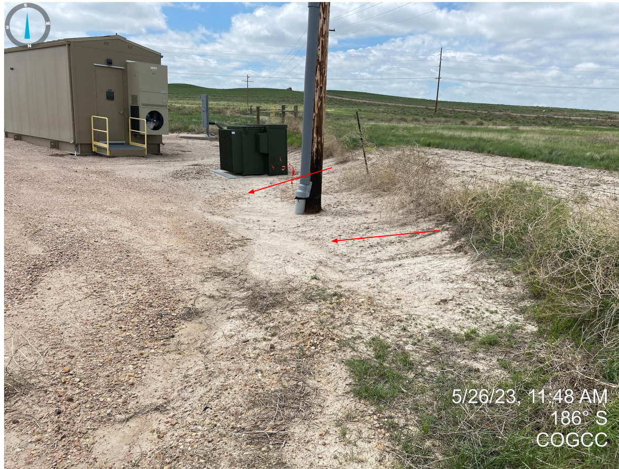
Photo 8. Western portion of location. Evidence of sediment transport onto the location from unstabilized bank/soils. Additional repair or implementation of stormwater BMPs is required to prevent further erosion from occurring.
