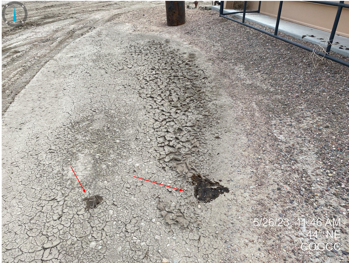
Photo 7. Stained soil will need to be properly cleaned and disposed of per Rule 905.e.
