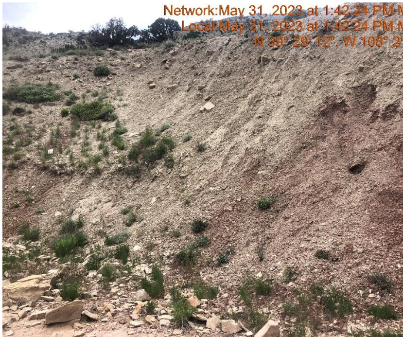
Photo #162 Cut slope lacks stabilization.
