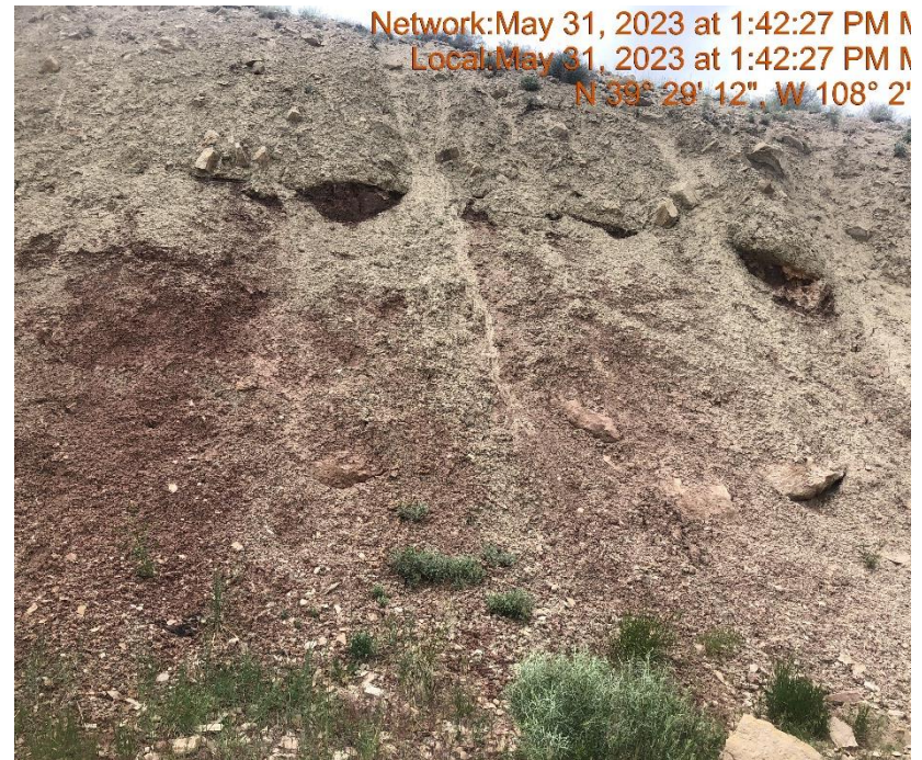
Photo #163 Cut slope lacks stabilization
