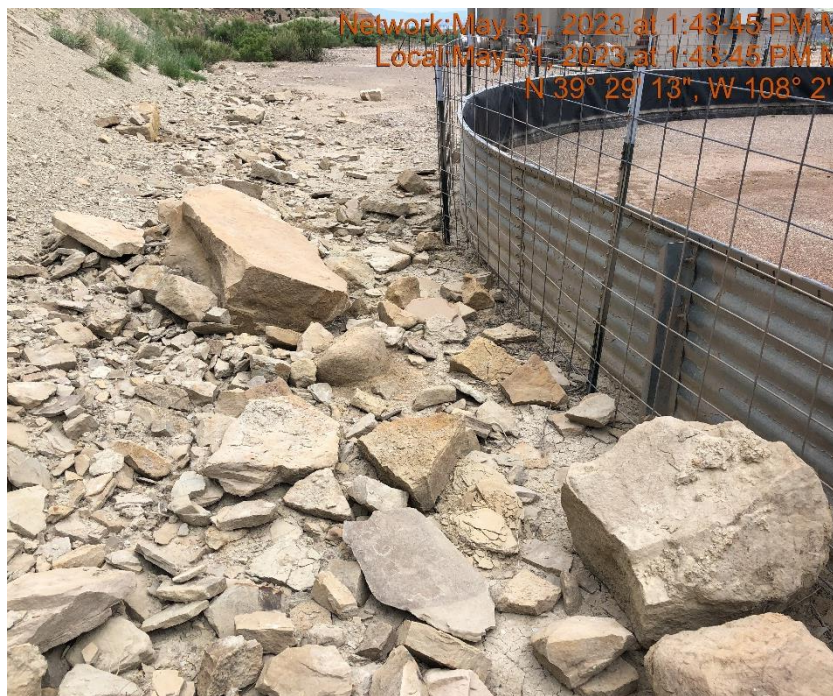
Photo #169 Rocks and sediment encroaching on tank containment.
