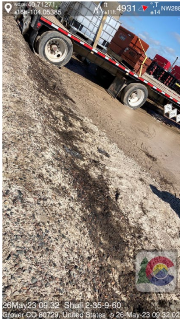
Photo 17 – Stained soil observed along locations earthen secondary containment berm - staining appears to be from previously observed impacts as noted Inspection Doc #708200264.
