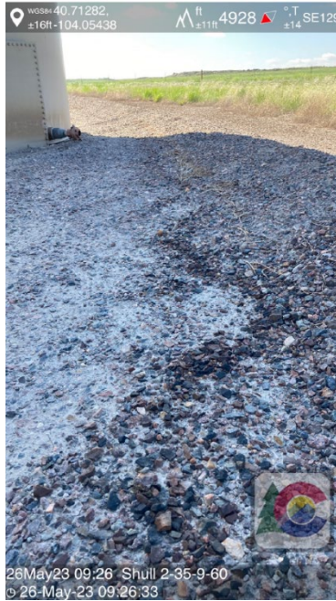
Photo 11 – Stained soil observed along locations earthen secondary containment berm - staining appears to be from previously observed impacts as noted Inspection Doc #708200264.
