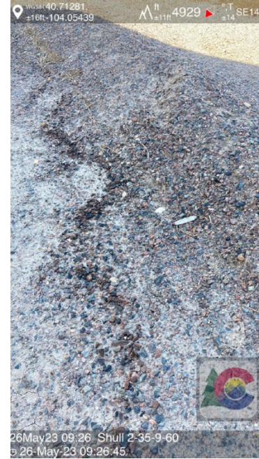
Photo 12 – Stained soil observed along locations earthen secondary containment berm - staining appears to be from previously observed impacts as noted Inspection Doc #708200264.
