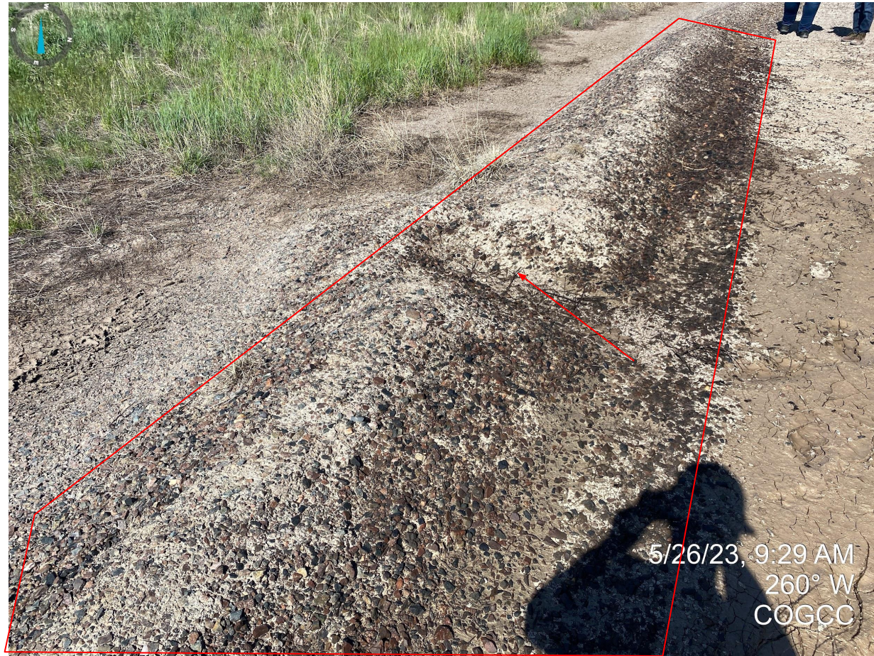
Photo 6. See comments in Photo 5. Hydrocarbon stained berm material pictured.
