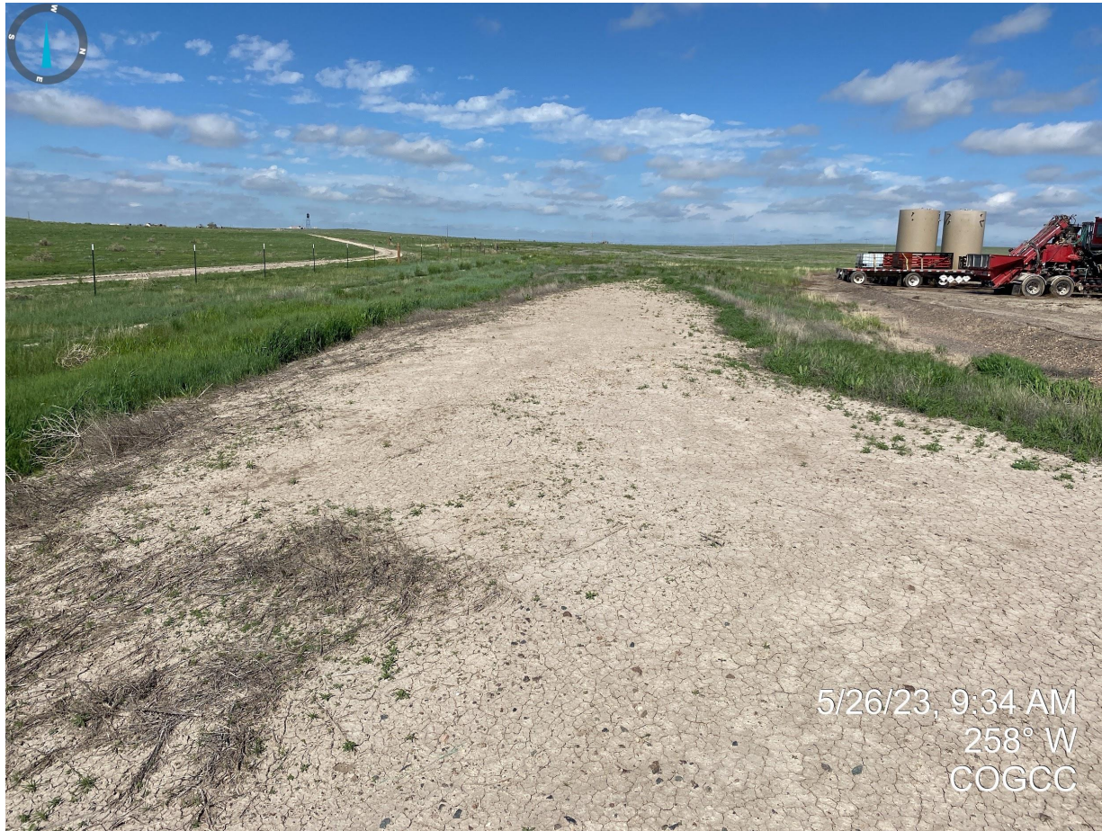
Photo 3. Topsoil stockpiles are predominantly bare soil with no evidence of uniform vegetation cover. Undesirable vegetation (e.g. kochia) was also observed growing in portions of the topsoil stockpile. Additional reclamation activities are required.
