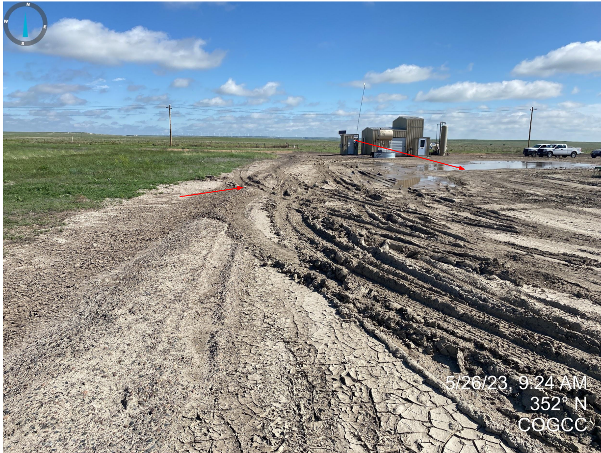
Photo 5. Stormwater BMPs do not appear to be properly functioning as stormwater is pooling throughout the location and leading to unstabilized production areas. Additionally, berm BMPs around the location are breached, have equipment parked on them, and are stained with apparent hydrocarbons.
