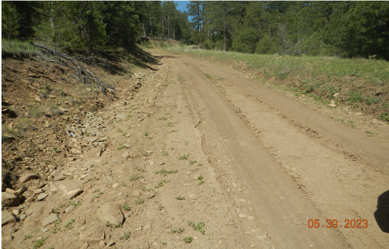
Photo 6. Facing west along the access road. Some of the rock check dams previously installed have washed out and there is insufficient BMP's to prevent erosion.
