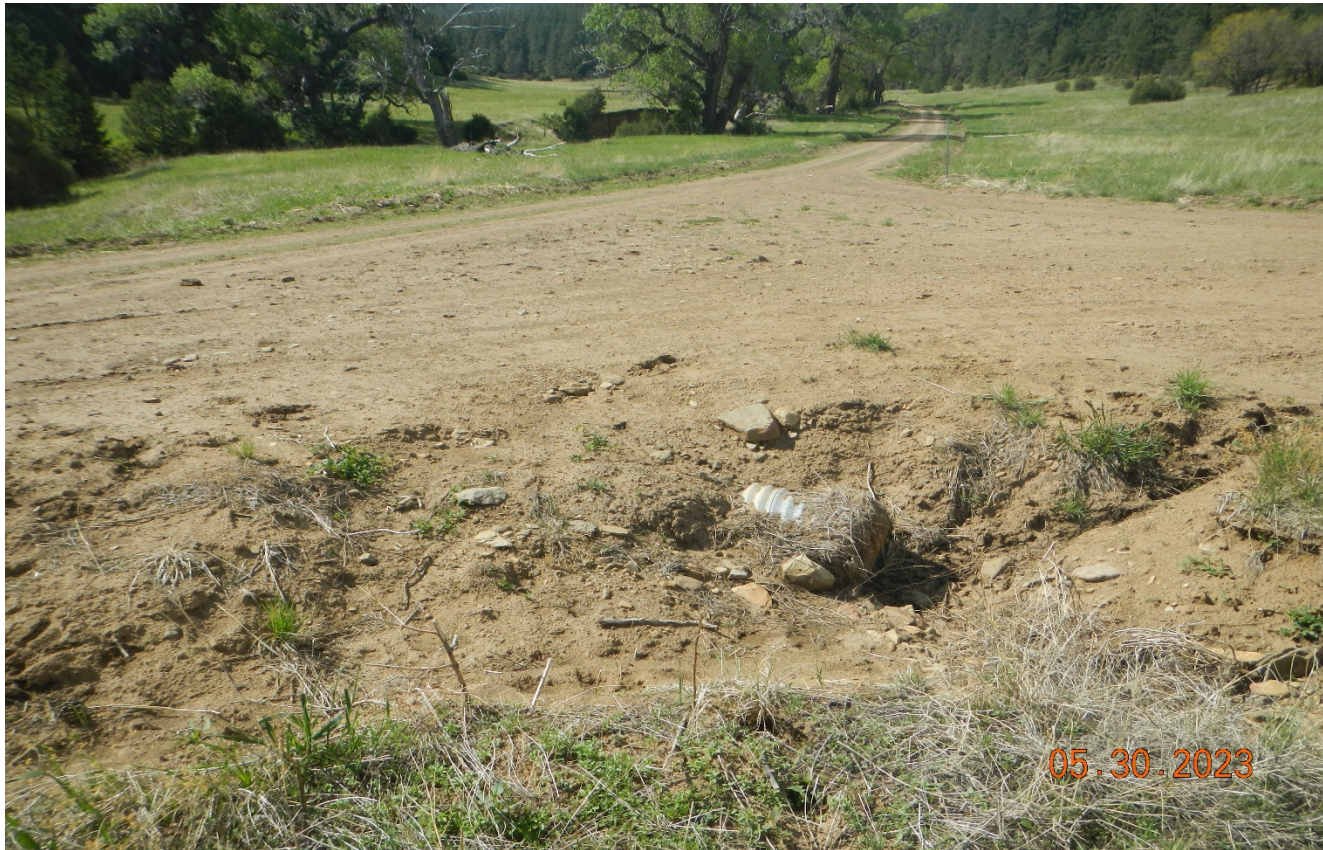
Photo 4. The culvert inlet is filled in with sediment and debris. It appears a larger culvert is needed at this area to handle stormwater coming off the road and drainage. Previous corrective action not completed.
