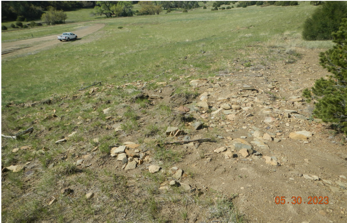
Photo 9. Facing south toward the run-on ditch which is filled in with sediment causing erosion of the cut slope. Previous corrective action is not completed.
