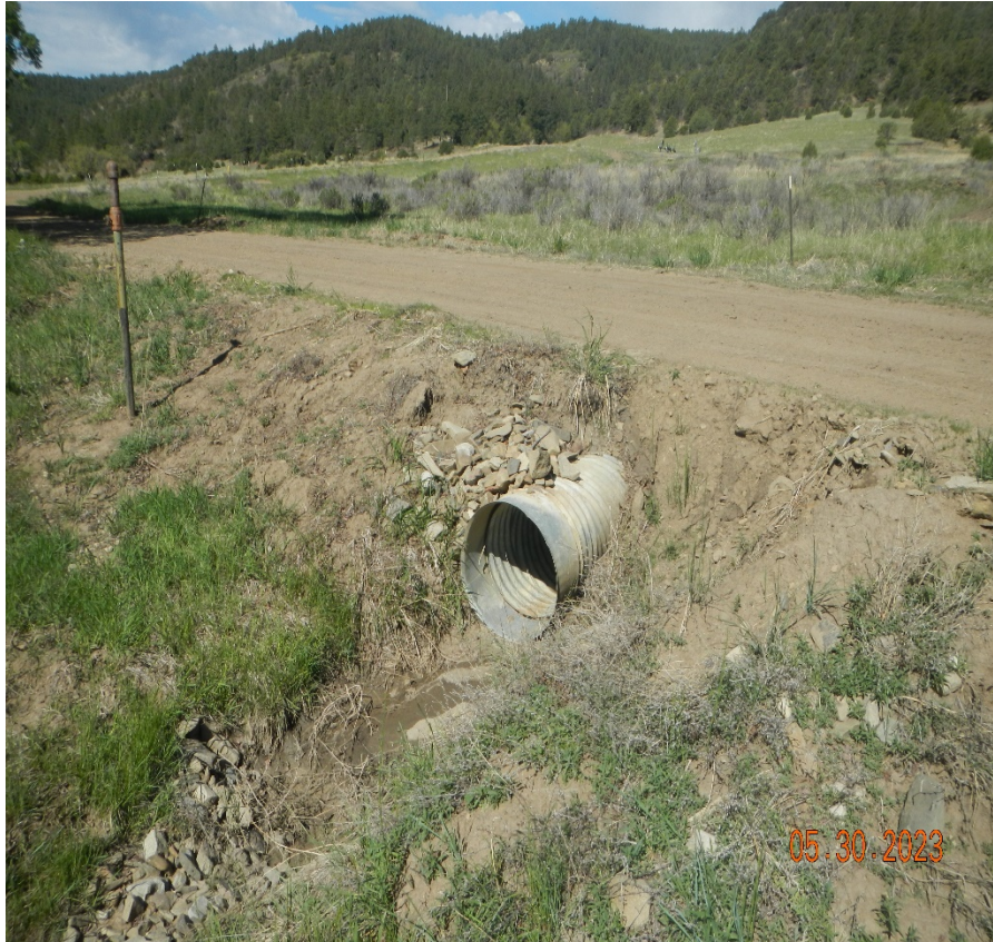
Photo 3. The next culvert along the road is also eroded at the culvert outlet with no outlet protection. Previous corrective action was not completed.
