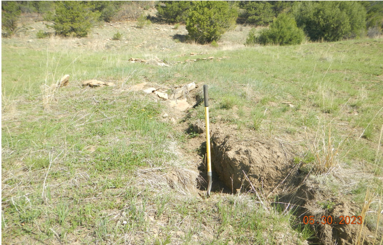
Photo 10. There are additional erosion channels along the south side of the location. Previous corrective action is not completed.
