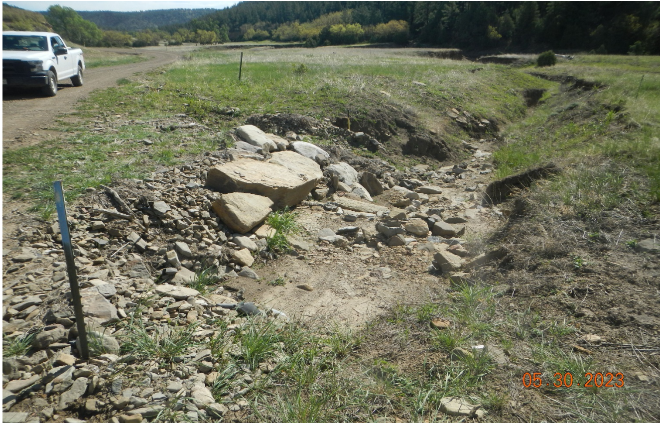
Photo 2. Facing toward the culvert outlet. The culvert outlet has eroded and needs to be repaired. Previous corrective action was not completed. BMP's must be installed per good engineering practice. (E.g. Rock outlet protection should include geotextile fabric)
