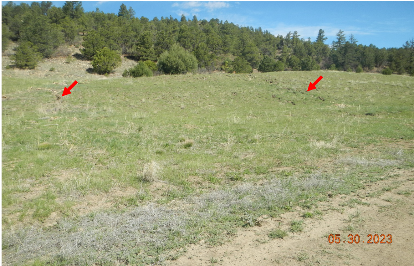
Photo 11. Facing north at the wellsite. Areas of erosion are visible at red arrows along the cut slope.
