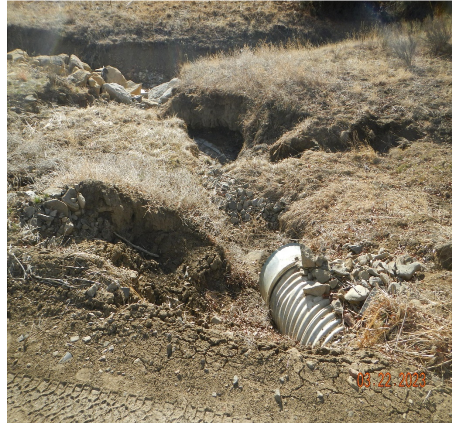
Photo 3. The next culvert along the road is also eroded at the culvert outlet with no outlet protection. Previous corrective action was not completed.
