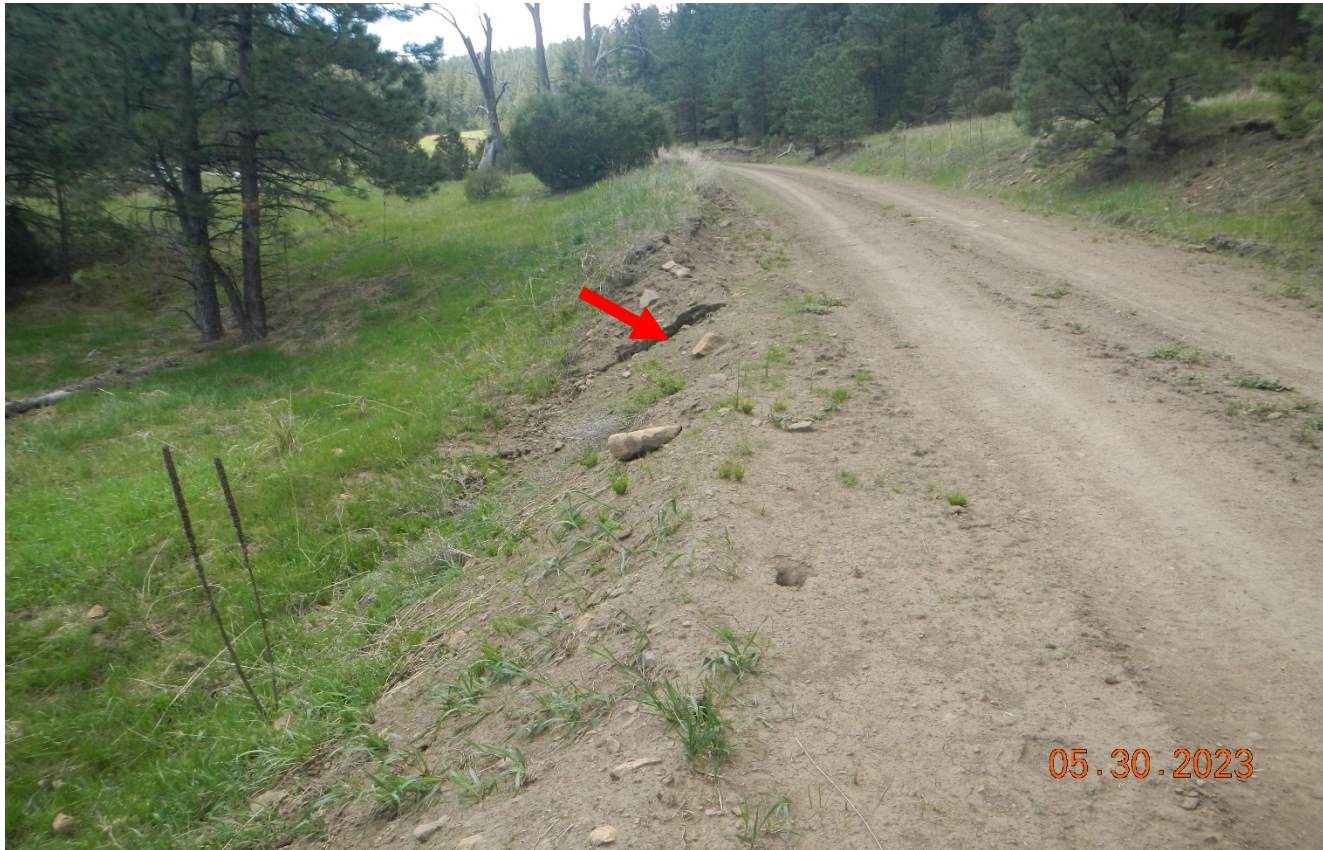
Photo 3. There was an erosion gully along the road that has been partially filled in however it was never stabilized. Erosion is beginning to occur in occur again which is transporting sediment into the stream drainage. Previous corrective action was not completed.
