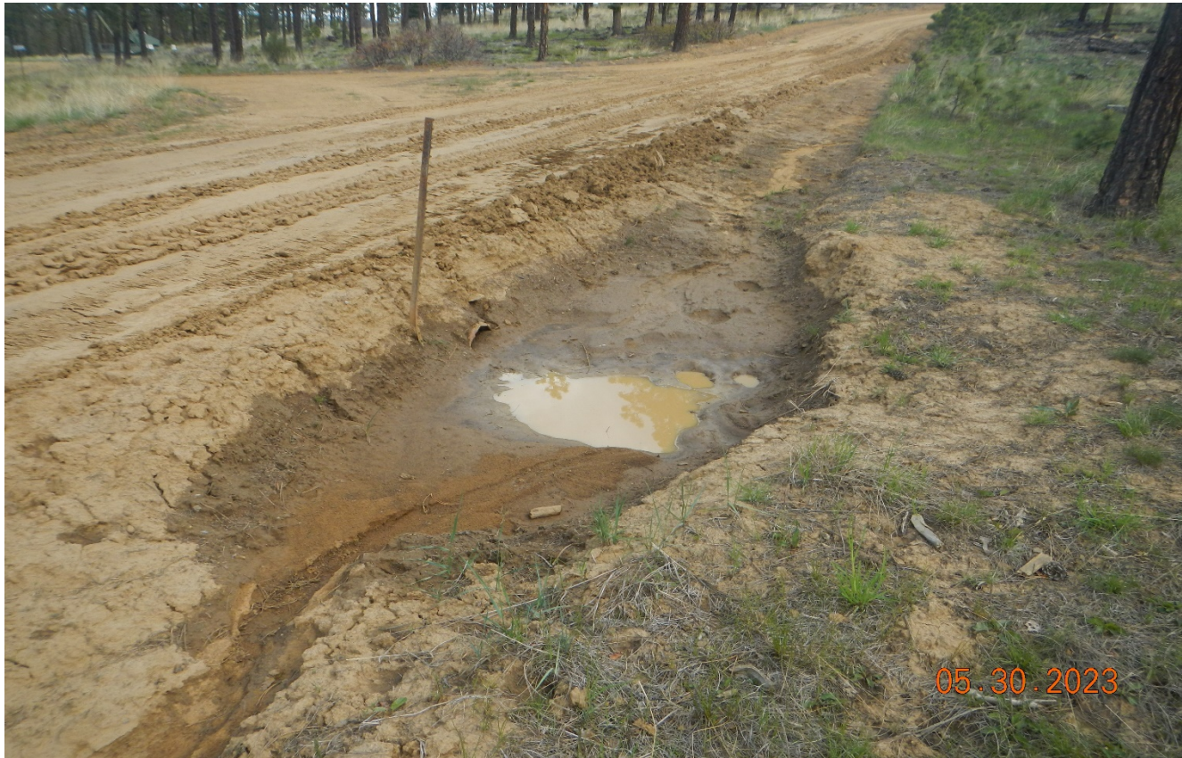
Photo 8. This culvert is full of sediment which needs to be cleaned out. Lat/Long:36.99405,-104.84710. Previous corrective action not completed.
