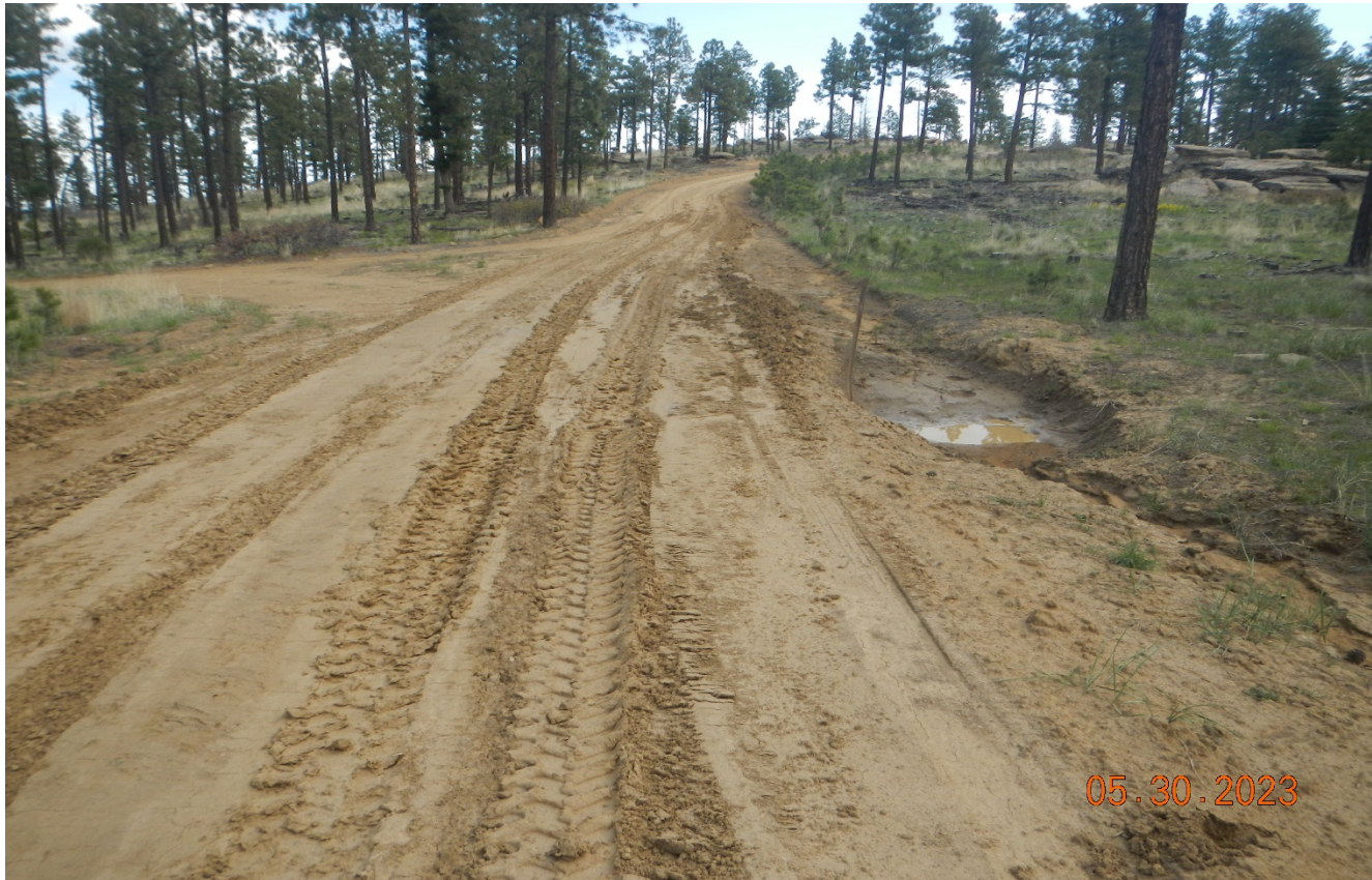
Photo 7. Facing northeast along the main access road. This culvert is filled in with sediment and stormwater is accumulating in this area causing erosion and vehicle tracking.
