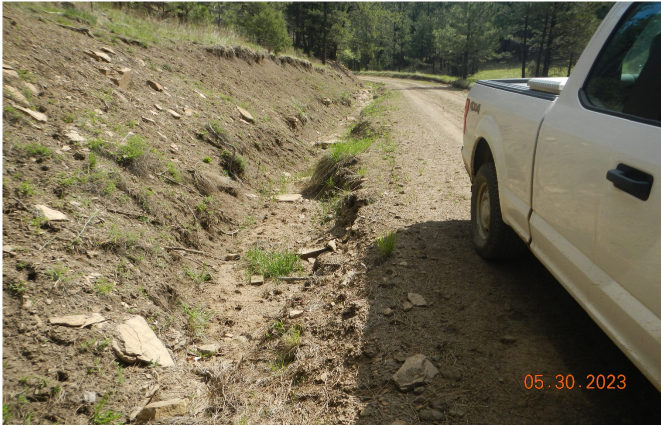
Photo 6. Further along the road near the Colorado line. The roadside and road is eroded and needs to be repaired and stabilized. Previous corrective action not completed.
