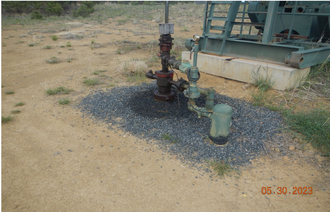
Photo 10. There is stained soil at the wellhead that needs to be cleaned up.
