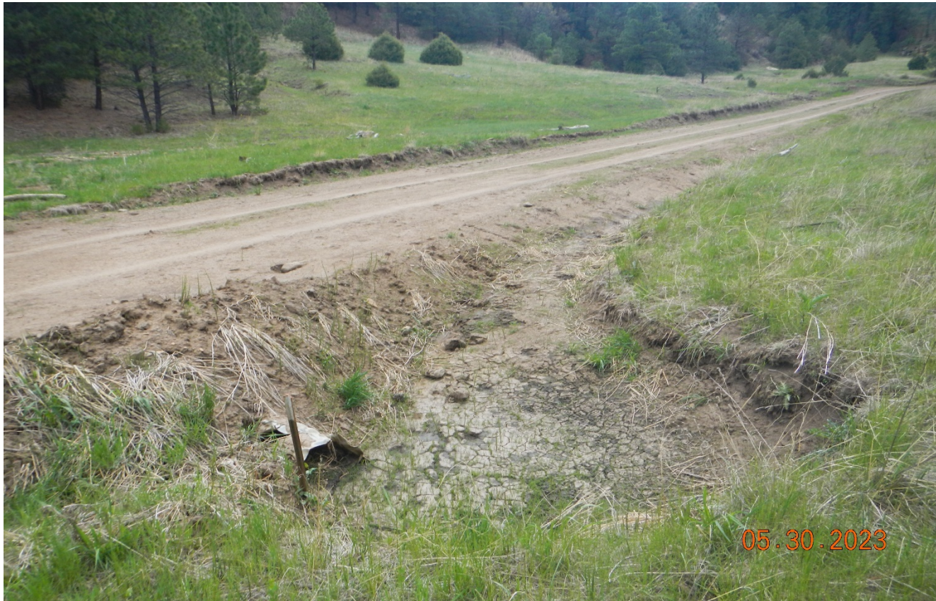
Photo 2. This culvert inlet was cleaned out by the Operator however, the culvert is full of sediment and the inlet has filled back in with sediment. Previous corrective action was not completed. Lat/Long:37.00581,-104.83861.
