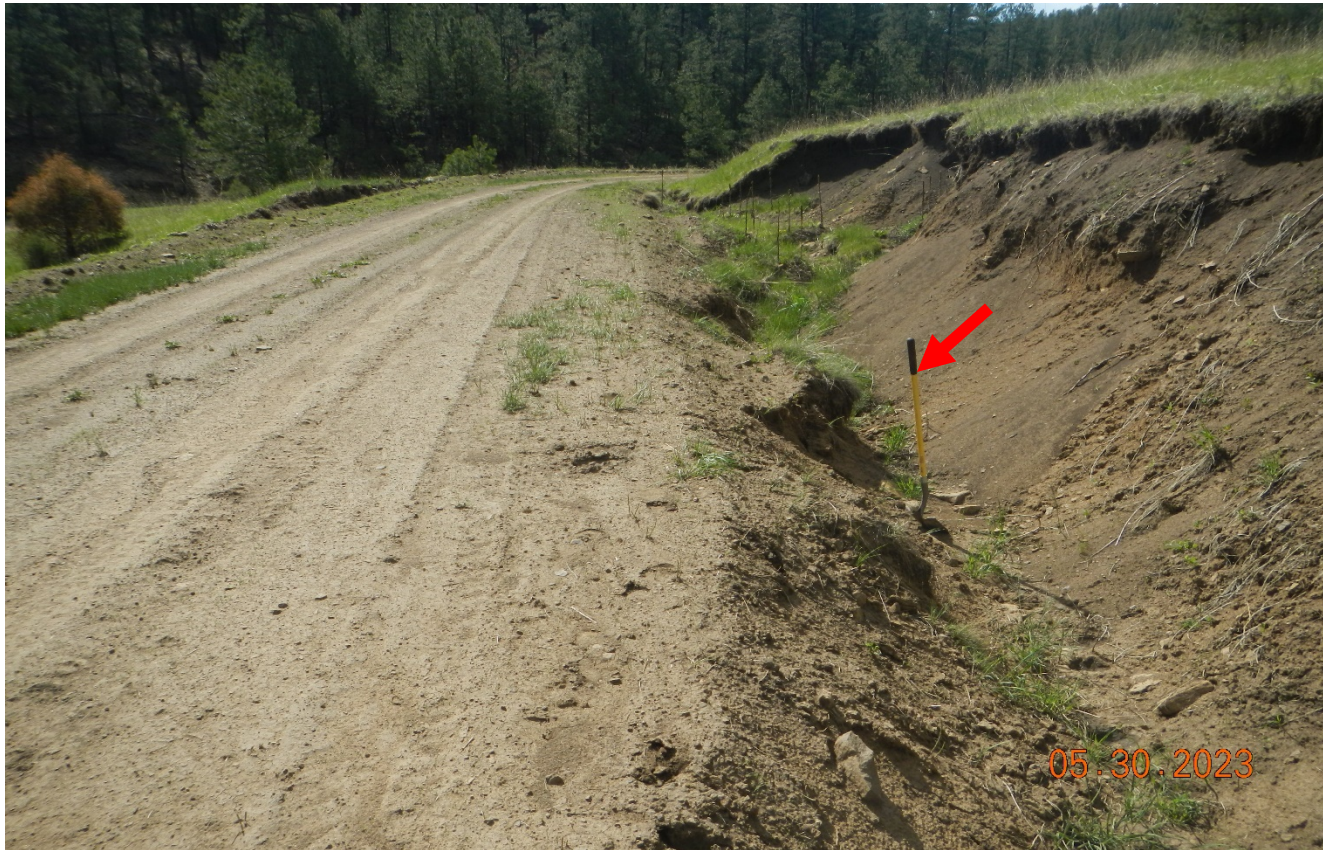
Photo 4. The side of the road is eroded and not stabilized. Erosion head cutting is continuing to occur further back into the slope. This area needs to be repaired and stabilized. Previous corrective action not completed. Red arrow points to 4.5 ft. shovel for scale. Lat/Long:36.99952,-104.83425.
