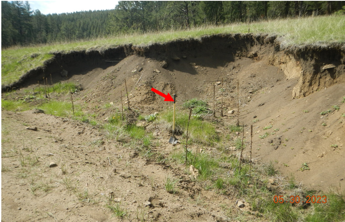
Photo 5. The side of the road is eroded and not stabilized. Erosion head cutting is continuing to occur further back into the slope. This area needs to be repaired and stabilized. Previous corrective action not completed. Red arrow points to 4.5 ft. shovel for scale. Lat/Long:36.99952,-104.83425.
