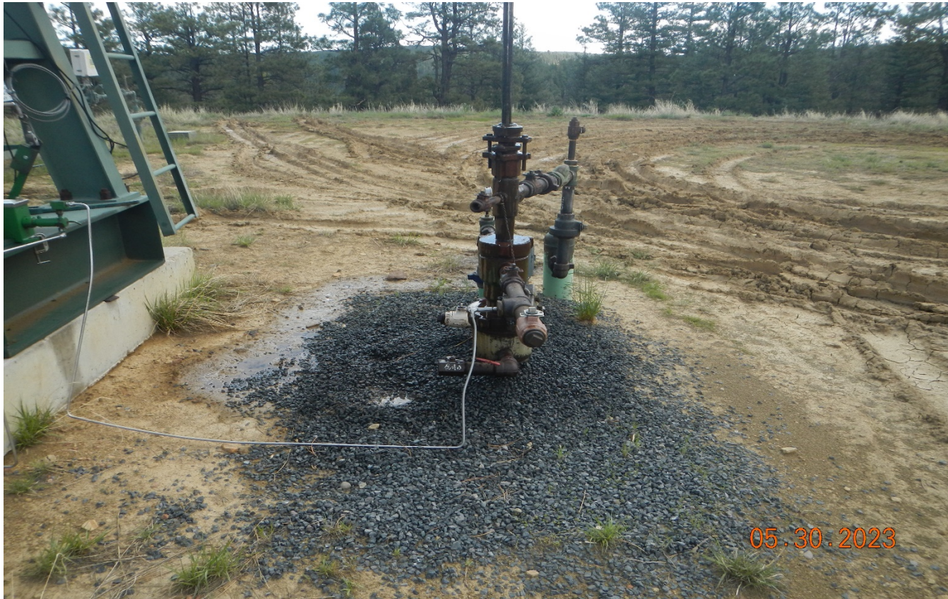
Photo 8. The wellhead is leaking and there are stained soils.
