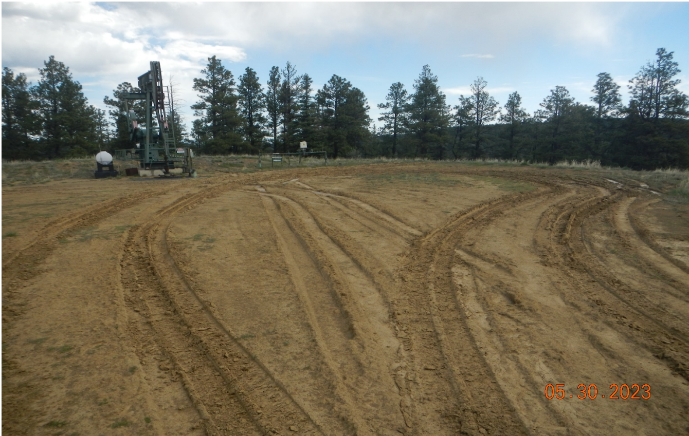
Photo 3. Facing northeast toward the wellsite. There is vehicle rutting at the location which is not stabilized to prevent vehicle tracking.
