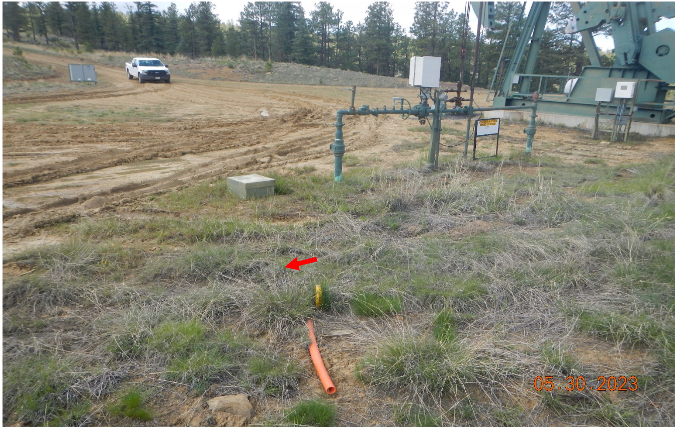
Photo 6. The guy line anchor marker has fallen over.
