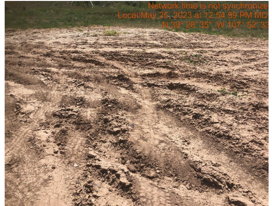
Photo #138 Location lacks stabilization.
