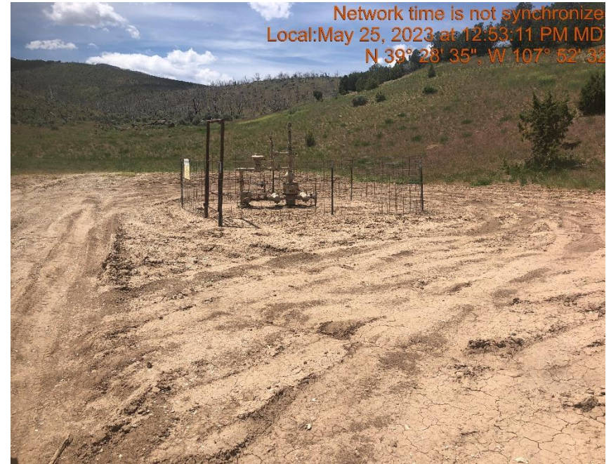
Photo #133 Location lacks stabilization.
