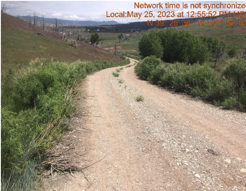
Photo #140 -Insufficient tracking BMP at entrance to location. To minimize the transport of sediment
