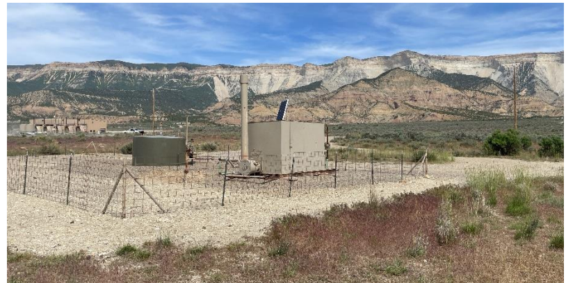
South East corner of location.
