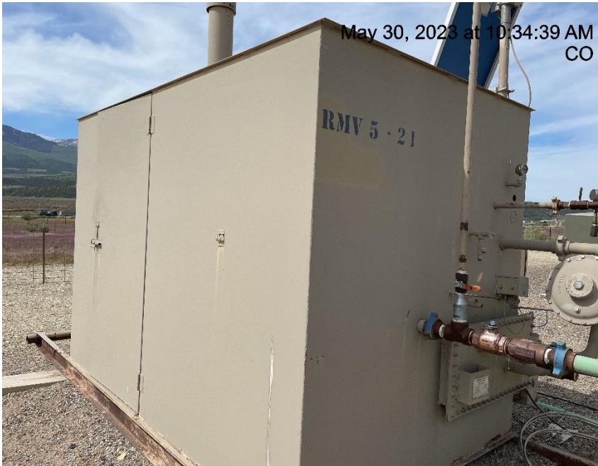
Photo # 9000 Meter calibration info not conspicuously posted
