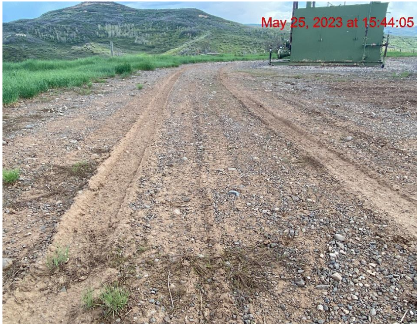
Location Lacks Stabilization – Photo #03928
