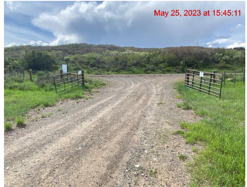
Insufficient Vehicle Tracking BMPs at Location Entrance/Exit – Photo #03929
