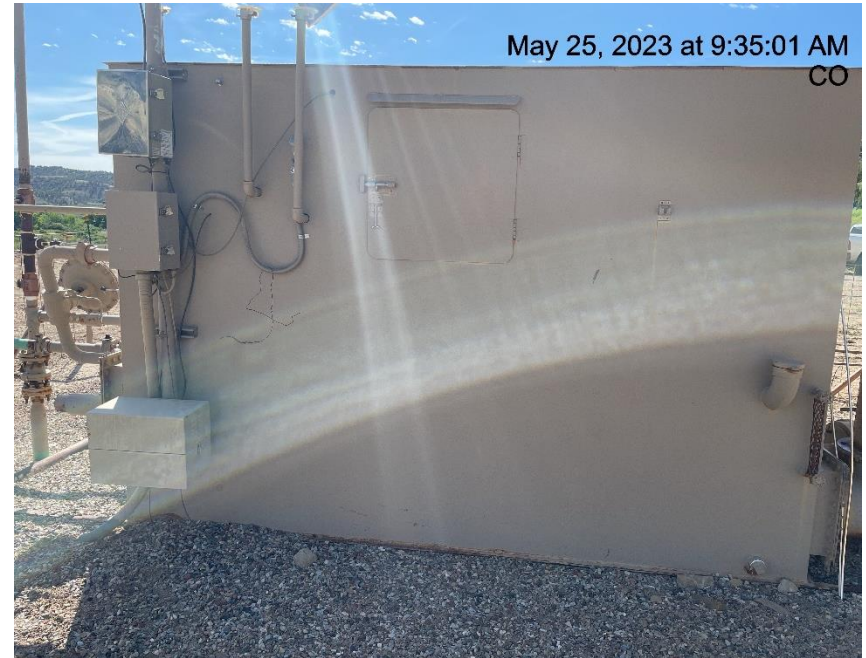
Photo # 8751 Meter calibration info not conspicuously posted
