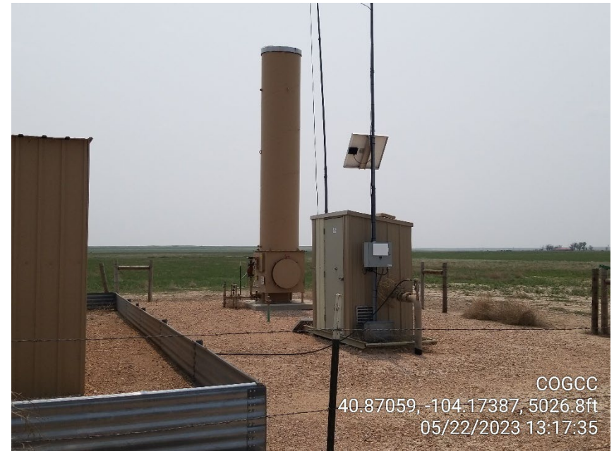
Photo 4 – ECD and Gas Meter
