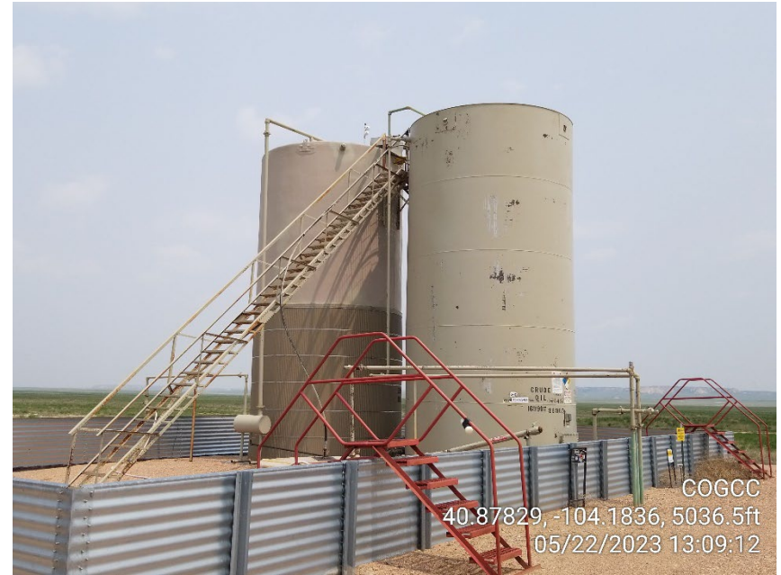
Photo 2 – Tank Battery
