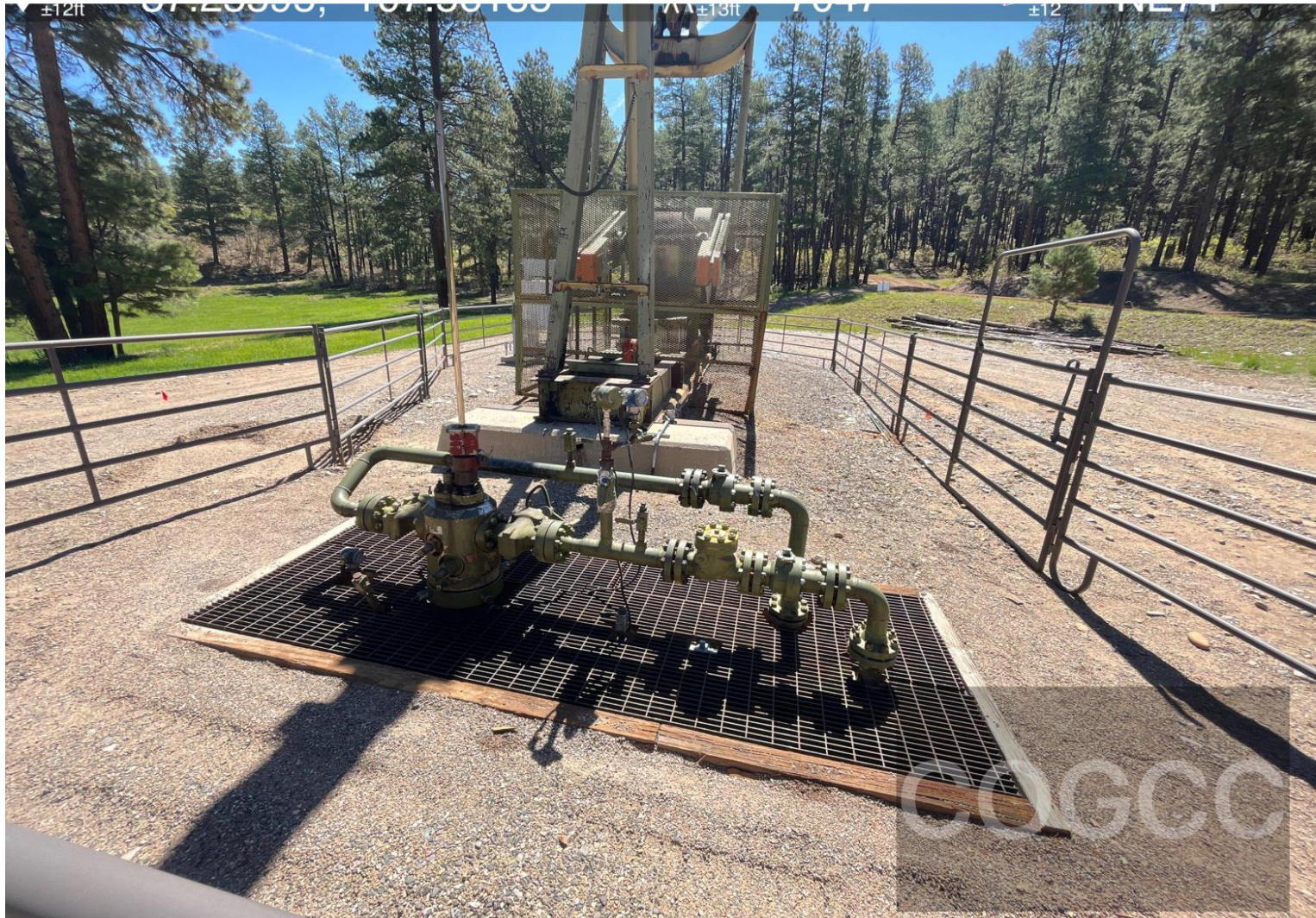
Photo #2 View of wellhead assembly.
