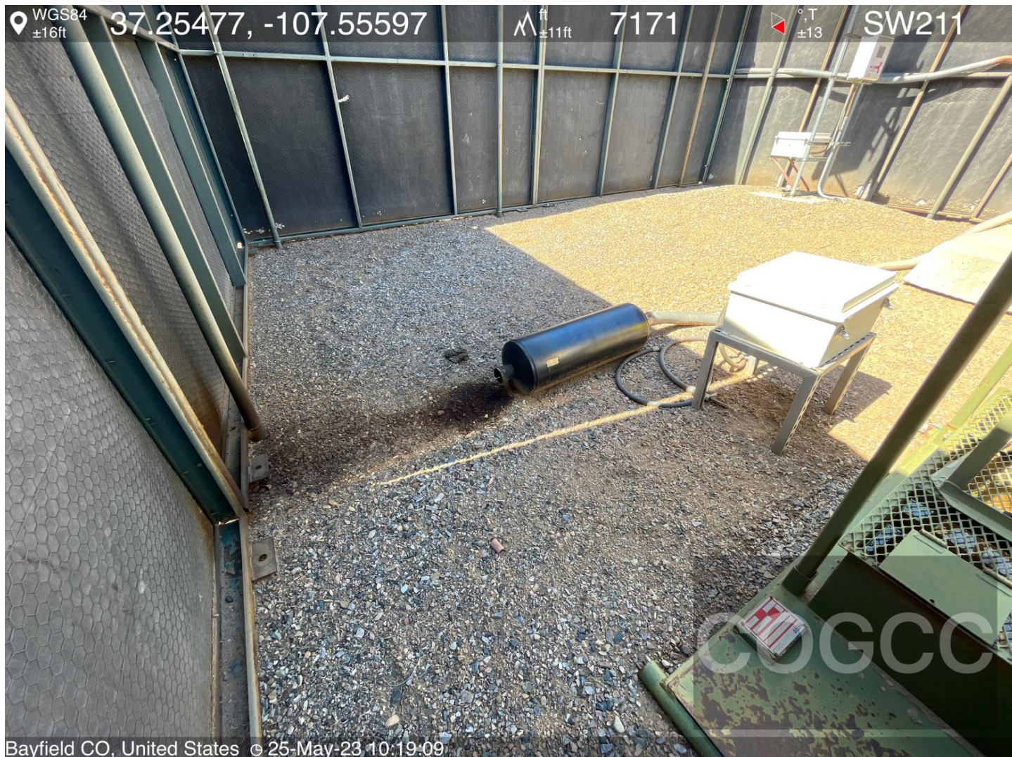
Photo #2 View of impacted material from exhaust muffler.
