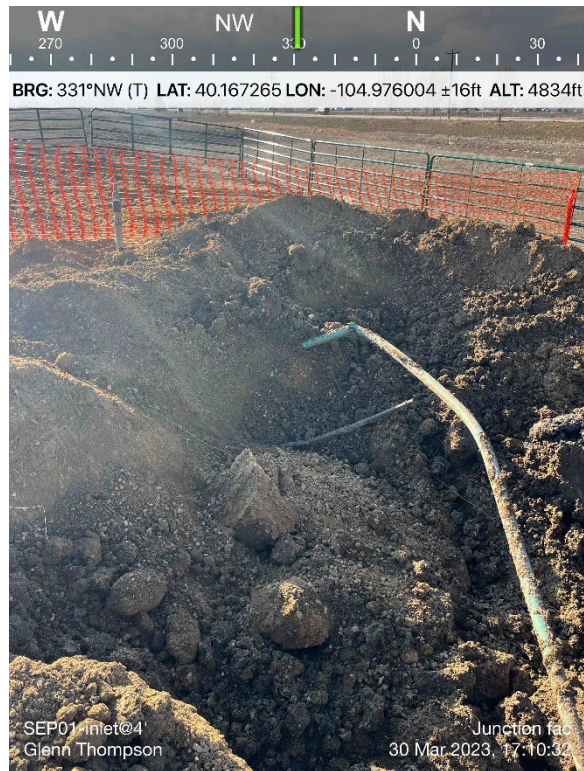
Separator Riser 01 Excavation
