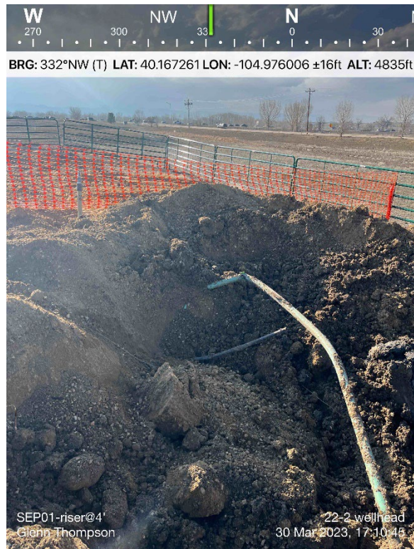
Separator Riser 01 Excavation
