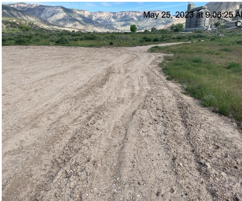
Photo # 8695 Lack of stabilization/compaction on location
