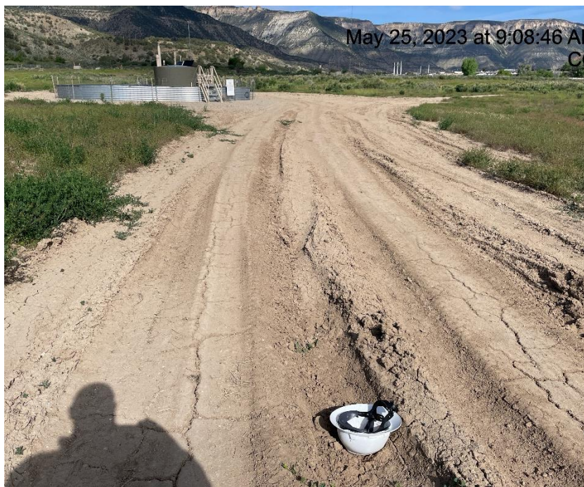
Photo # 8701 Lack of stabilization/compaction on access road
