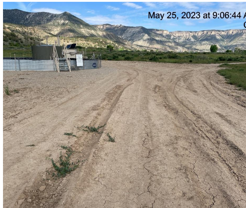
Photo # 8696 Lack of stabilization/compaction on location
