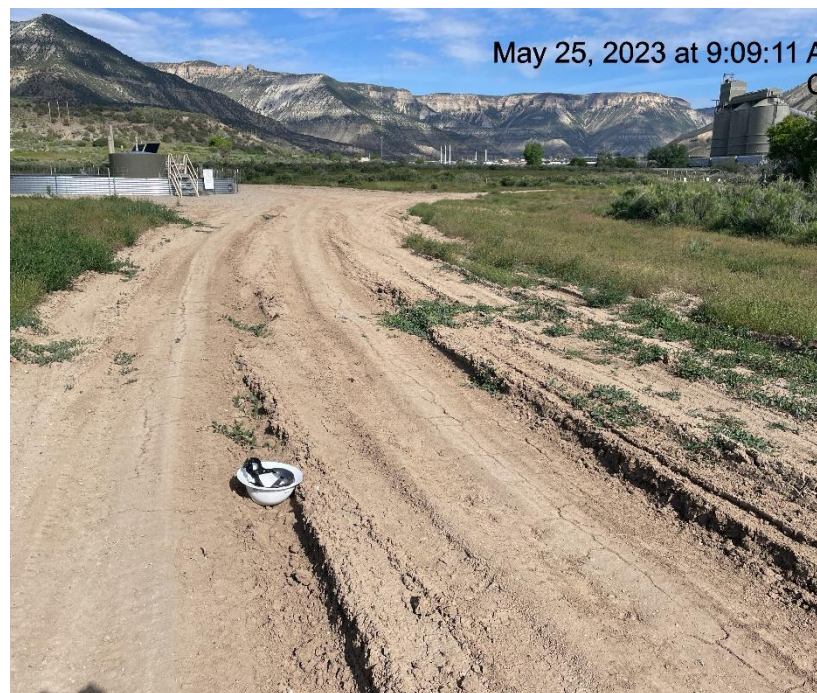
Photo # 8702 Lack of stabilization/compaction on access road
