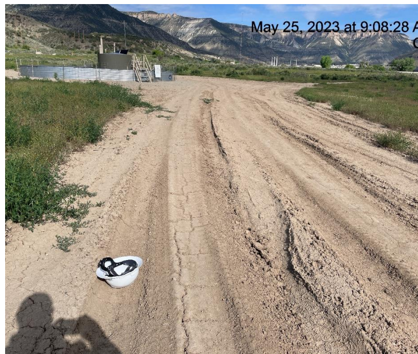
Photo # 8700 Lack of stabilization/compaction on access road
