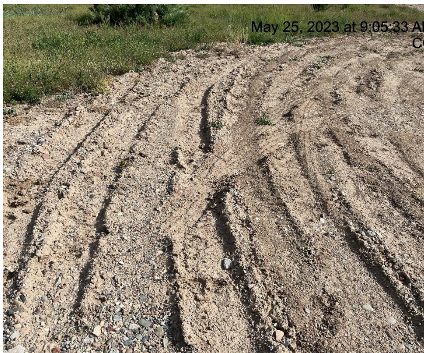
Photo # 8693 Lack of stabilization/compaction on location
