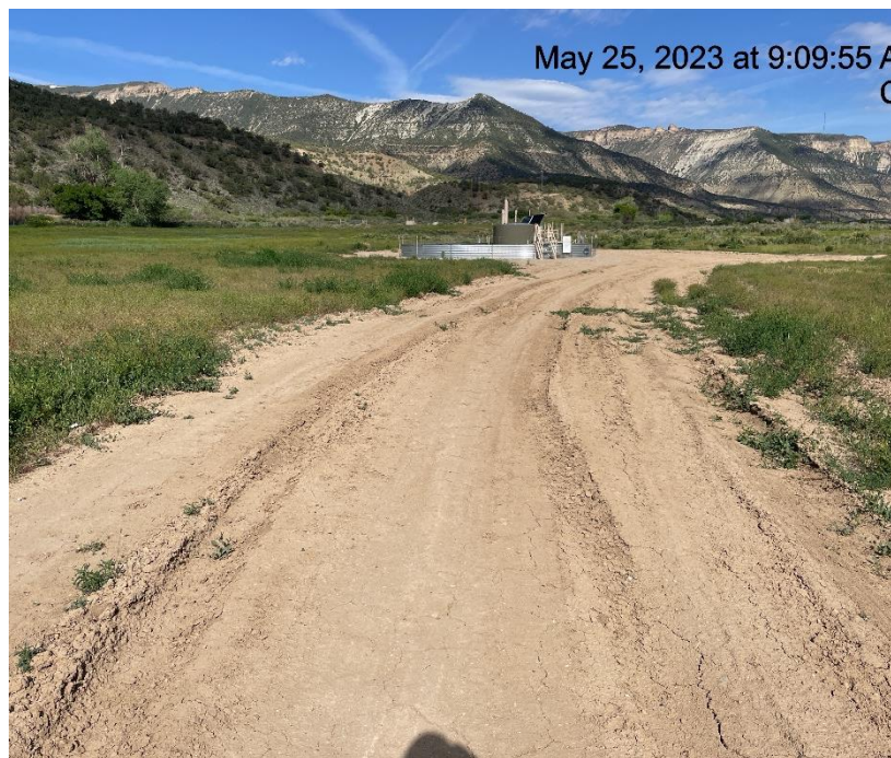
Photo # 8704 Lack of stabilization/compaction on access road
