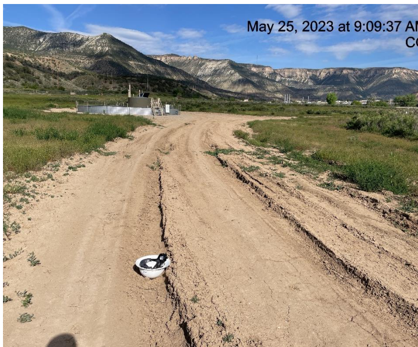
Photo # 8703 Lack of stabilization/compaction on access road
