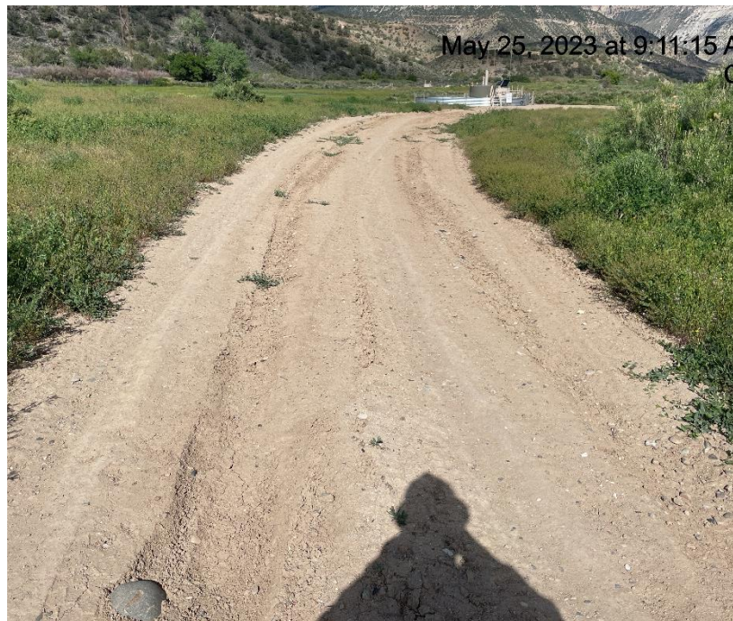
Photo # 8706 Lack of stabilization/compaction on access road
