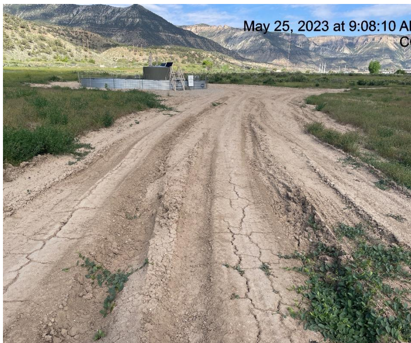
Photo # 8699 Lack of stabilization/compaction on access road
