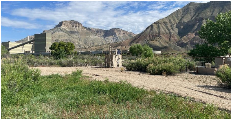
South West corner of location.
