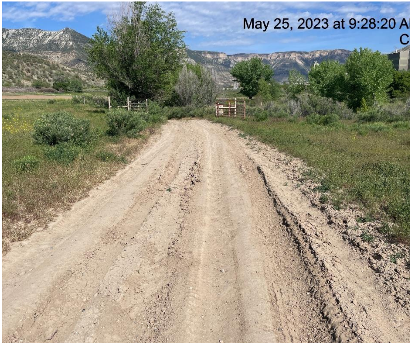
Photo # 8740 Lack of Stabilization/Compaction on spur road
