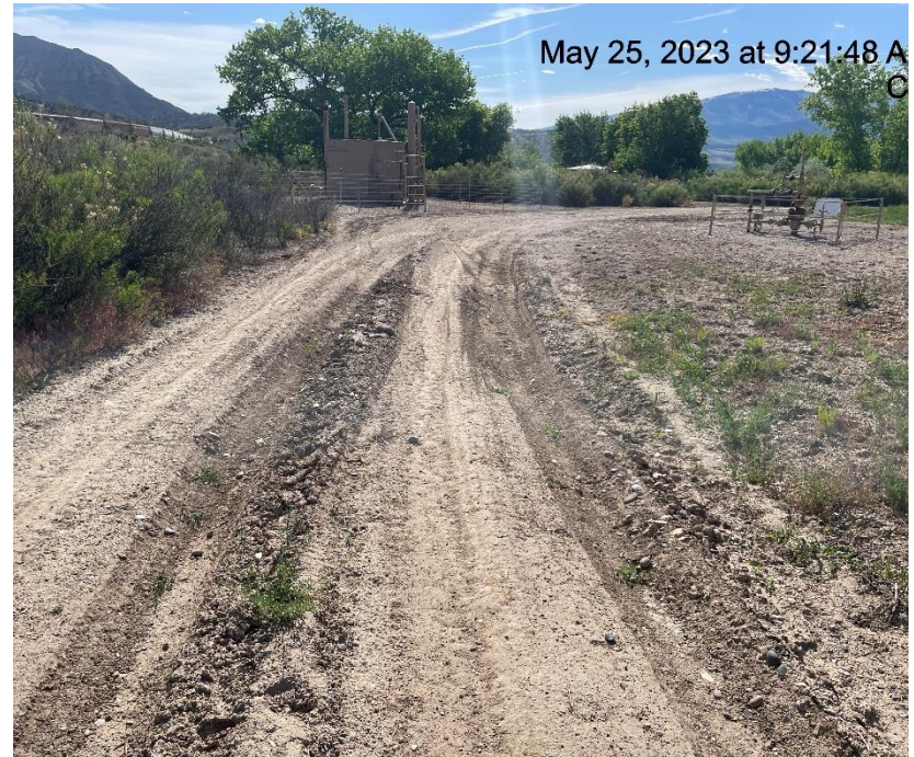
Photo # 8721 Lack of Stabilization/Compaction on location
