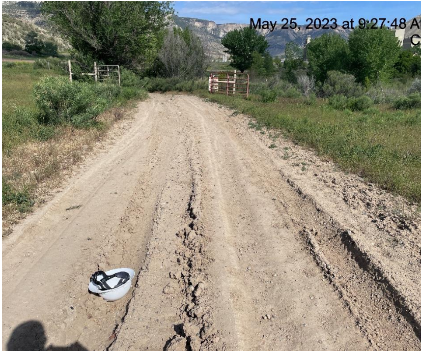
Photo # 8738 Lack of Stabilization/Compaction on spur road
