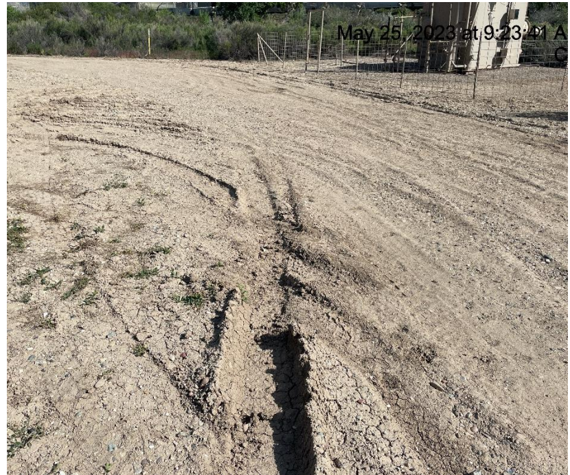
Photo # 8730 Lack of Stabilization/Compaction on location
