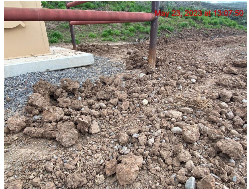
Site Degradation/Transportation of Sediment – Photo #03862
