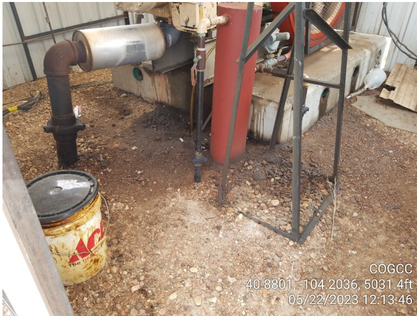
Photo 5 – Stained Soil at Gas Engine
