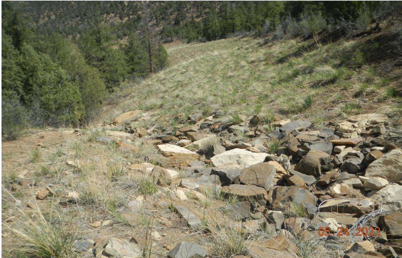
Photo 4. Facing north along the reclaimed road. There is rock rip/rap installed in the drainages.
