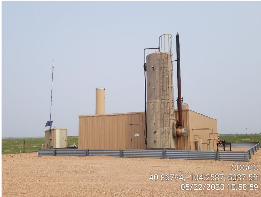
Photo 7 – Heater Treater, Gas Meter and ECD
