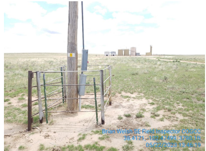
2. Electric panel on REA pole not secured to pole. Fence is installed around REA pole.
