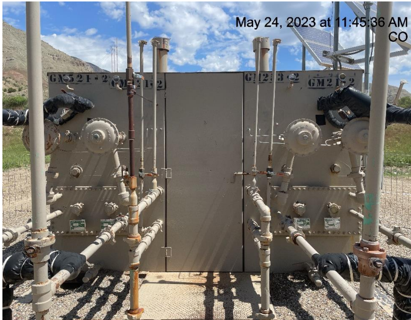
Photo # 8509 Meter calibration info not conspicuously posted
