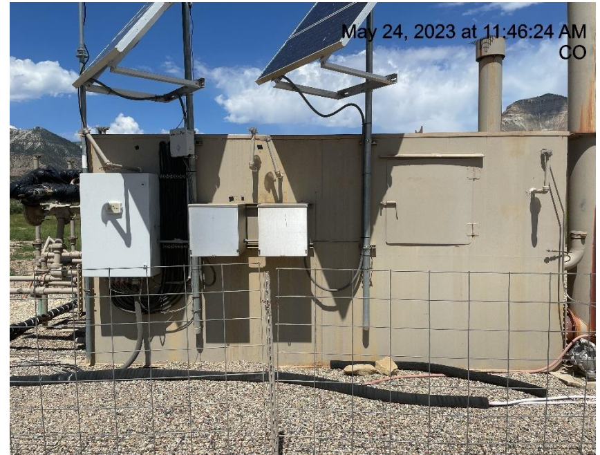
Photo # 8512 Meter calibration info not conspicuously posted
