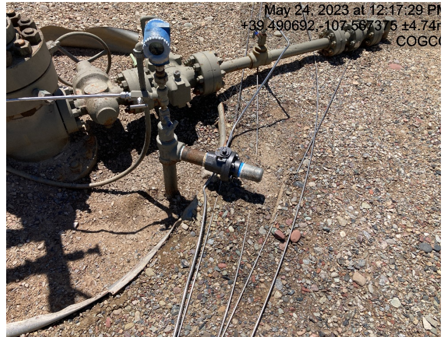
Follow up photo of new valve on Braden head
