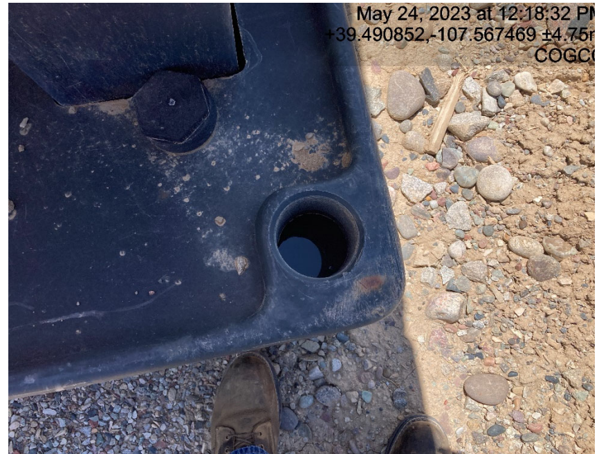
Follow up photo of chemical tank containment still full of fluid.
