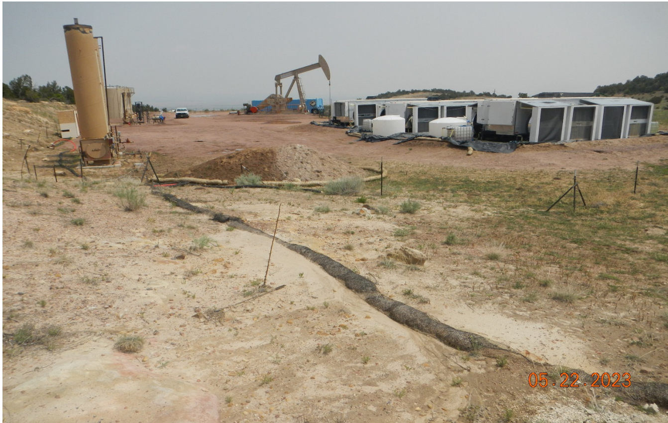
Photo 8. South side of the location facing northeast. The old wattles in this area need to be replaced or removed.
