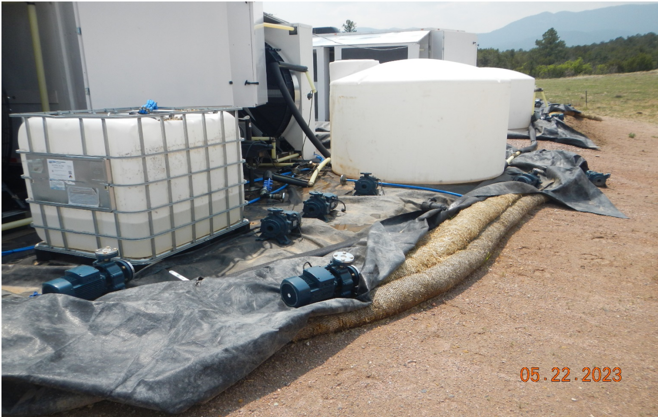
Photo 10. The plastic liner has become folded over needs to be repaired. There are water pump used to hold down the liner and should be removed if not need. Liner should be properly staked down.
