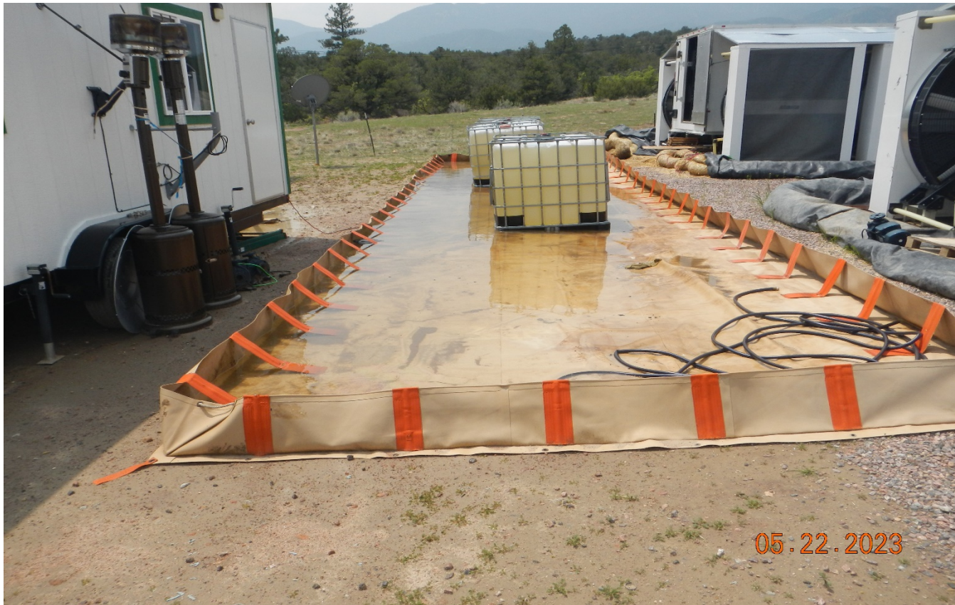
Photo 6. There is a portable secondary containment installed for the 2 chemical totes. The water needs to be removed to allow appropriate freeboard containment.
