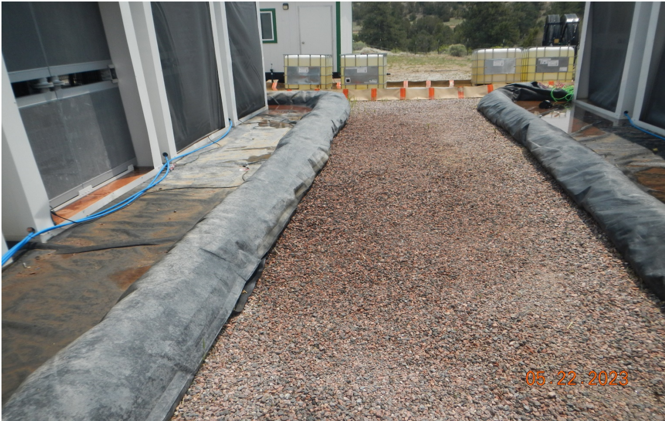
Photo 11. It appears in between the equipment there is darkened gravel from a possibly leak.
