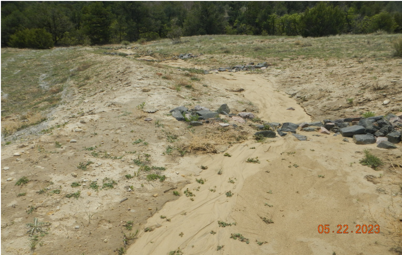
Photo 9. Facing south at the perimeter ditch. The check dams have filled in with sediment and need to be cleaned out.
