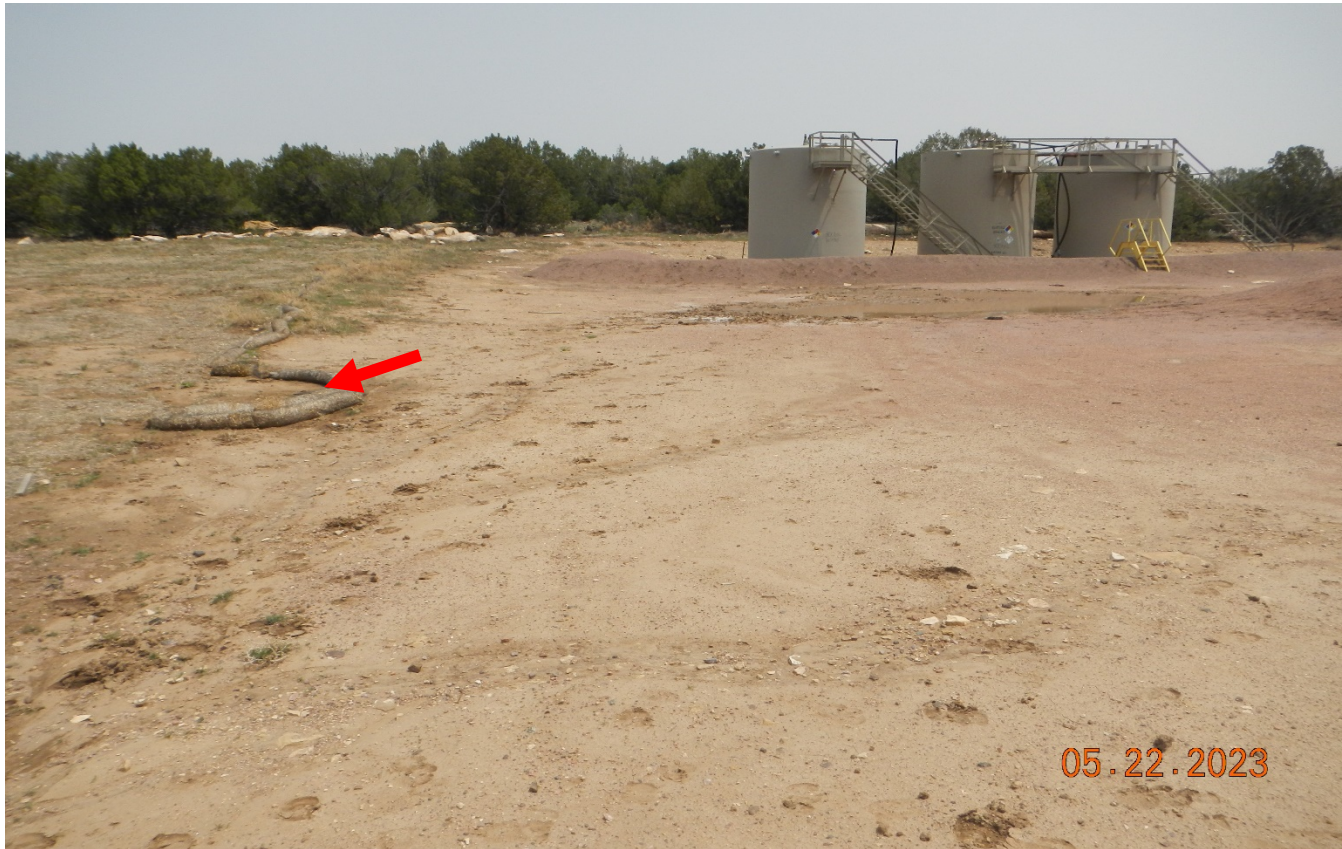
Photo 5. Facing north toward the location. There are displaced wattles that need to be repaired.
