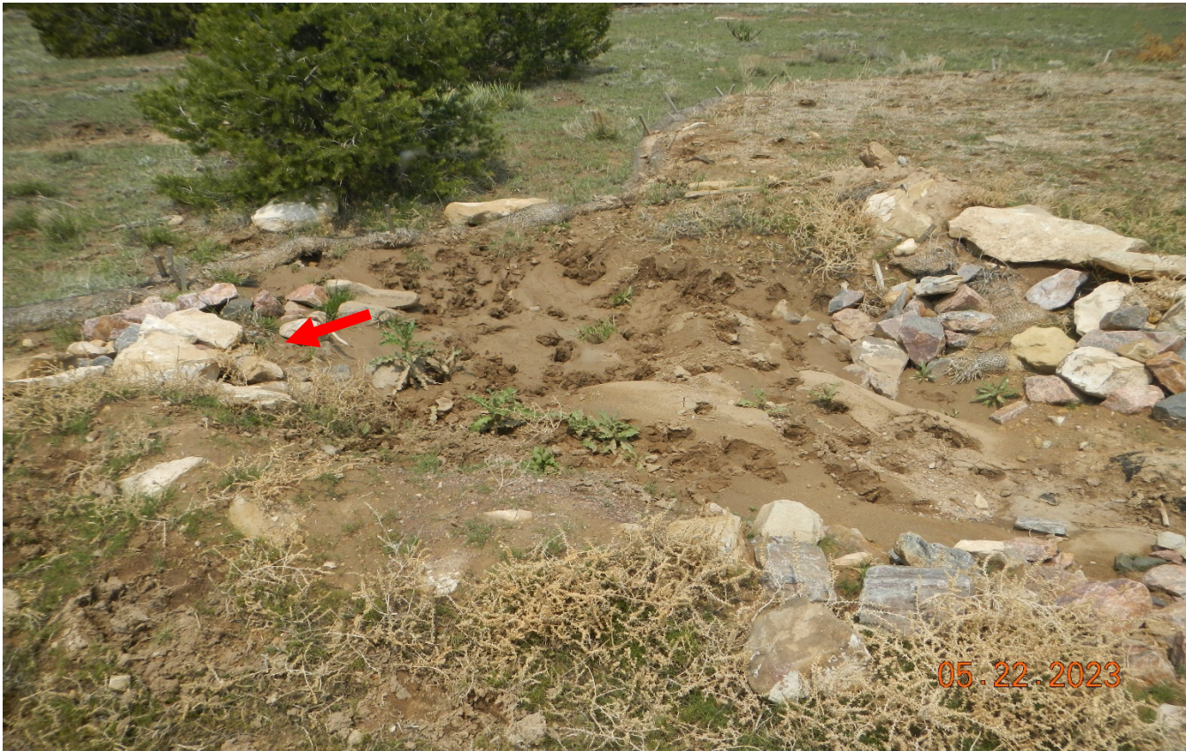
Photo 6. The sediment trap at the west side of the location has filled in with sediment and needs to be cleaned out. There are also noxious weeds (Canada thistle) that need to be controlled.
