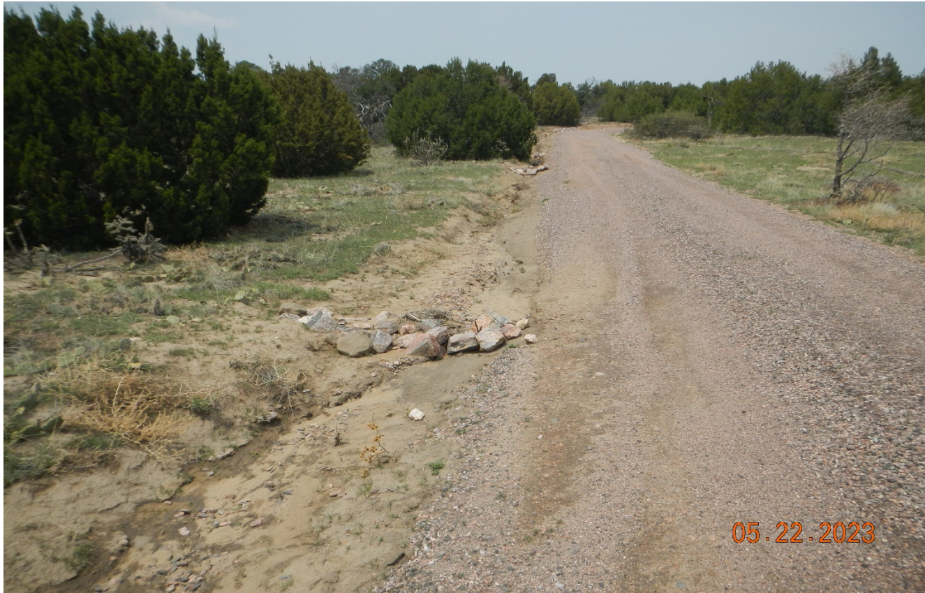
Photo 2. Facing northwest along the access road. There are some check dams where stormwater is going around the check dam. BMP maintenance is needed.
