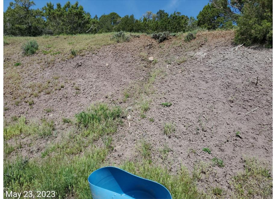
**Photo 3:** Photo shows slopes remain predominantly bare and exposed soils. Slopes lack stabilization and erosion degradation is evident.
