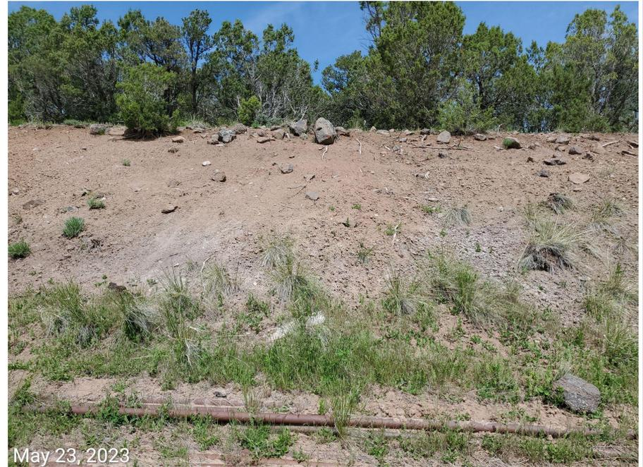
**Photo 2:** Photos 2-4 taken from the cut slopes of the Location. Photo shows slopes remain predominantly bare and exposed soils. Slopes lack stabilization and erosion degradation is evident.
